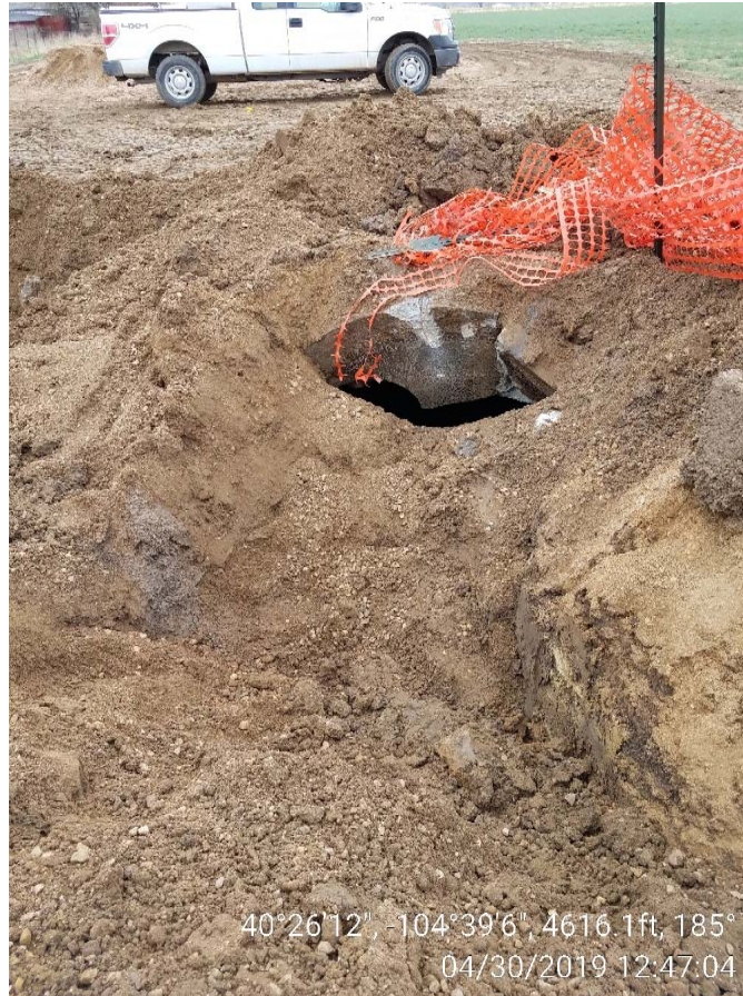
Photo 1 – Uncovered buried concrete produced water vessel.
