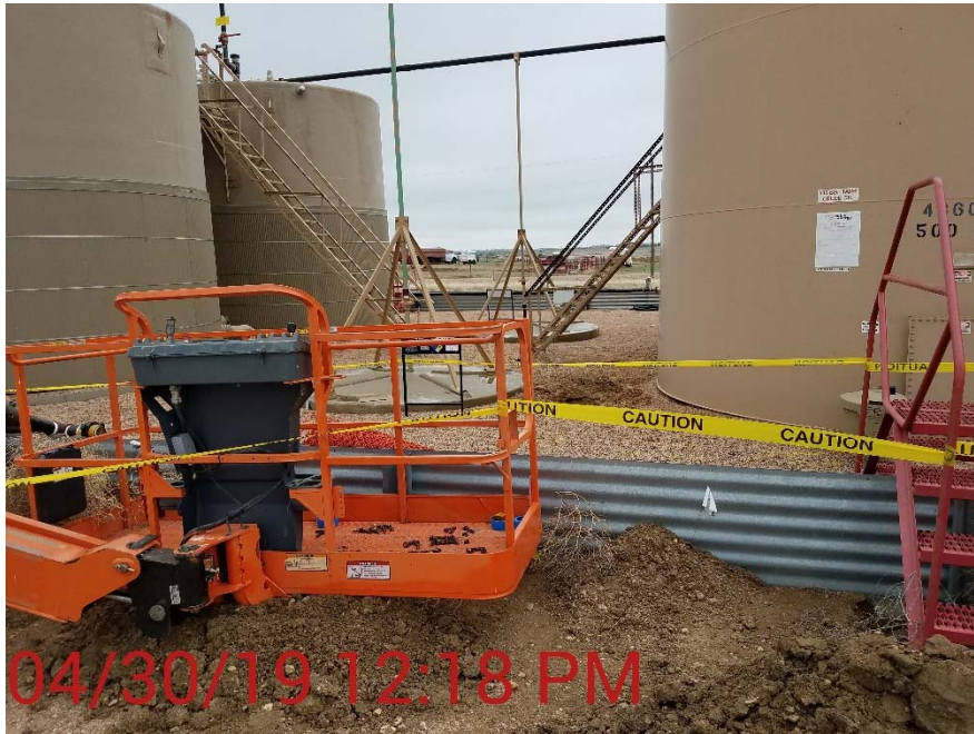
Photo 1 – Potholes/investigation near buried produced water vessel within non-lined secondary containment.
