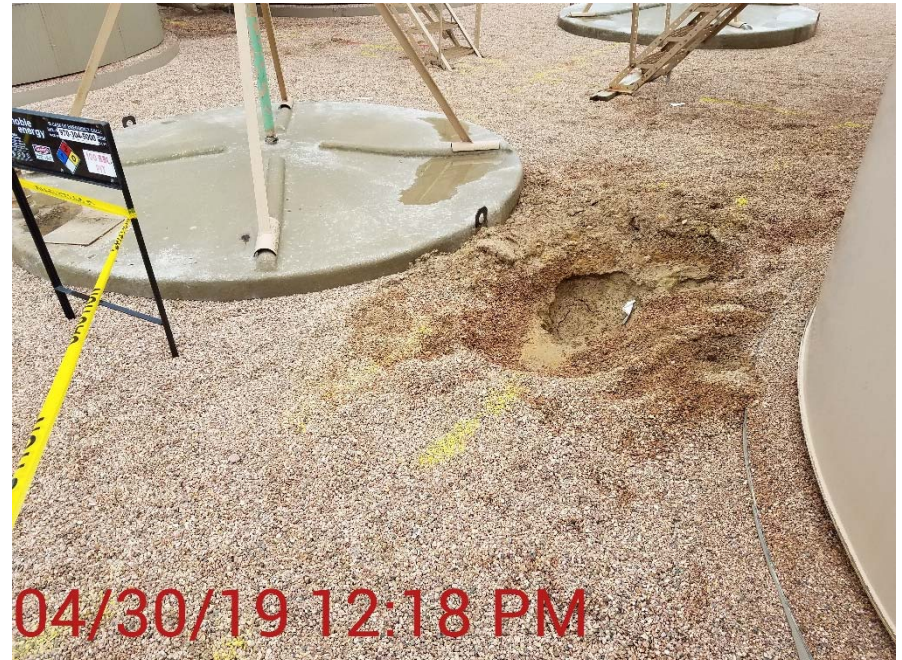
Photo 2 - Potholes/investigation near buried produced water vessel within non-lined secondary containment.
