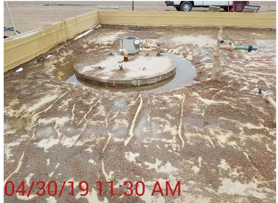
Photo 2 – Buried concrete produced water vessel within tank battery secondary containment.
