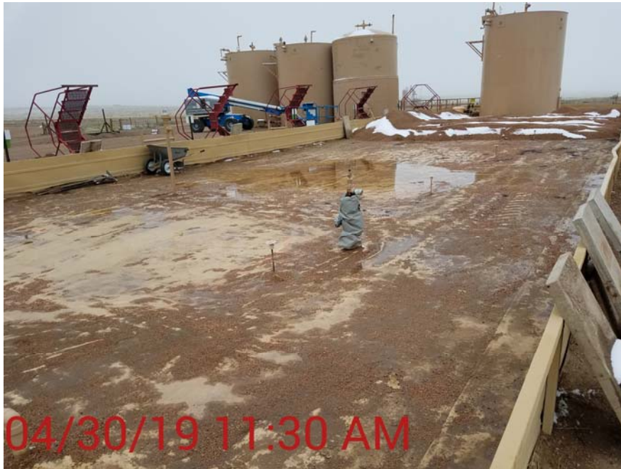
Photo 1 – View of dismantled tank battery with liner present.
