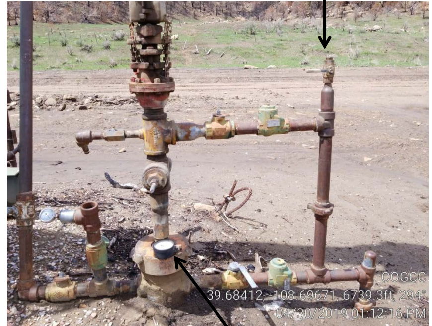
Photo 3. Gas leak at well head. Gage was attached on 10/3/2018 where gas leak is now occurring.
