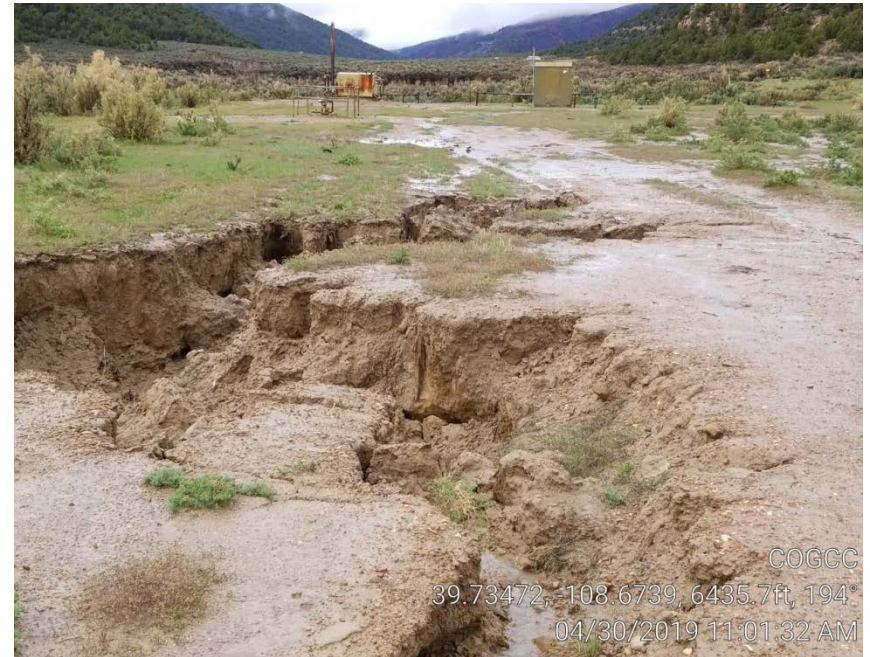
Photo 3. Erosion channel on edge of location.
