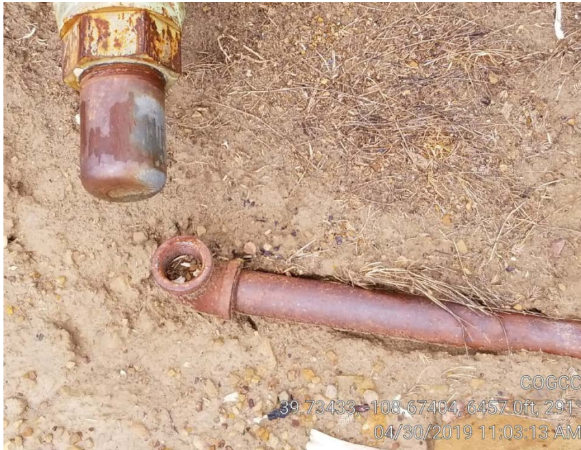
Photo 2. Uncapped riser next to wellhead.
