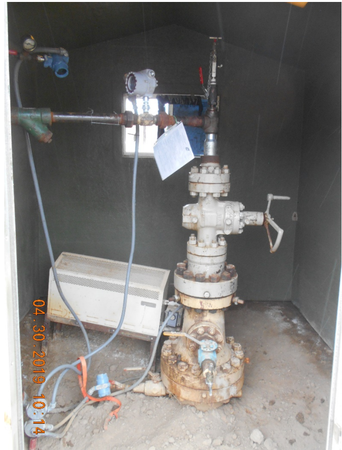
Wellhead inside housing
