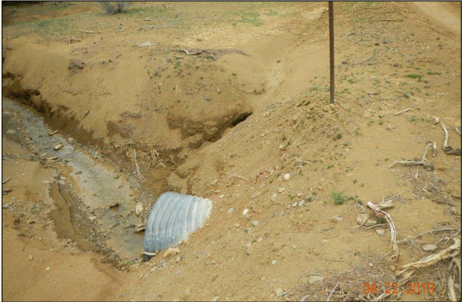
Photo 5. View of culvert inlet along the access road that is not stabilized. Runoff from the road flows into the stream and is not sufficiently managed.
