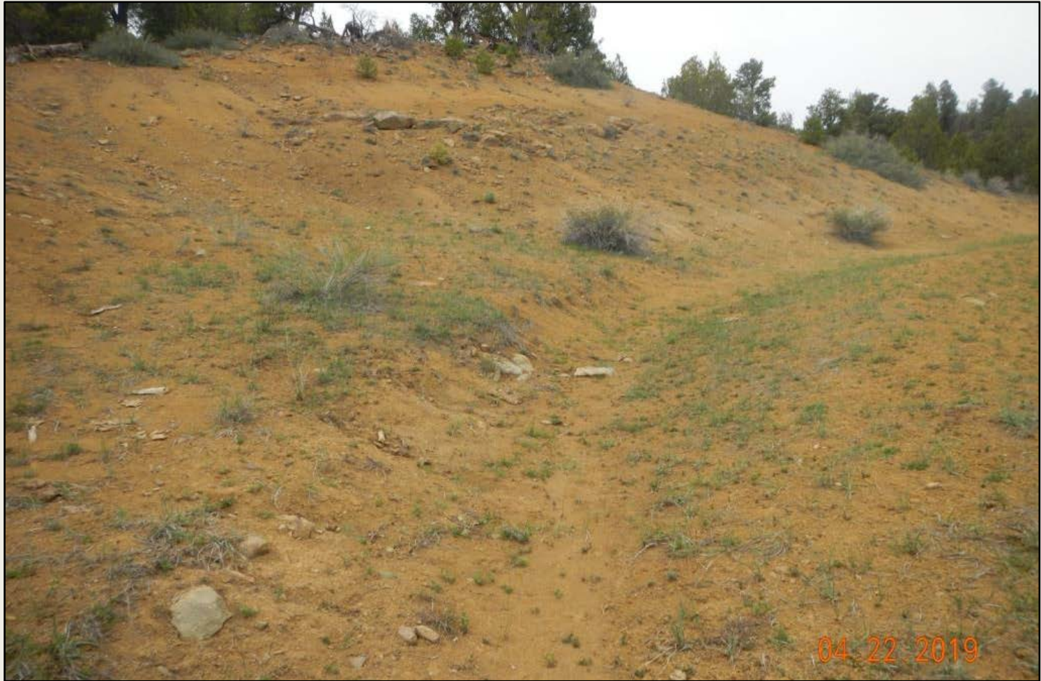
Photo 3. View of the southwestern cut-slope that is not stabilized
