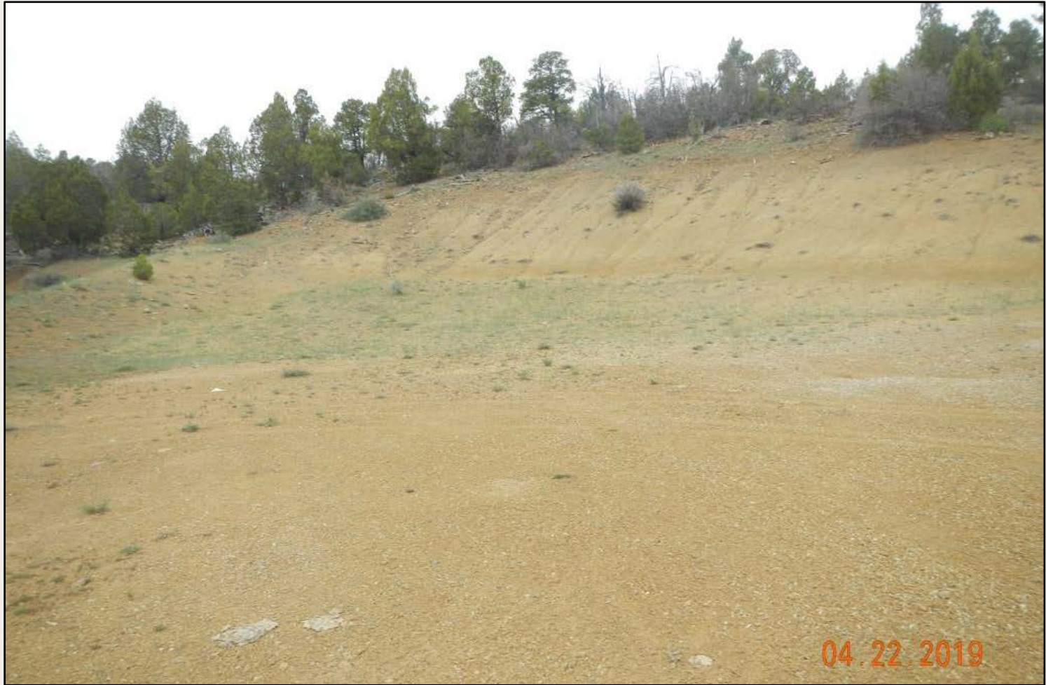
Photo 4. View of the northwestern cut-slope that is not stabilized.
