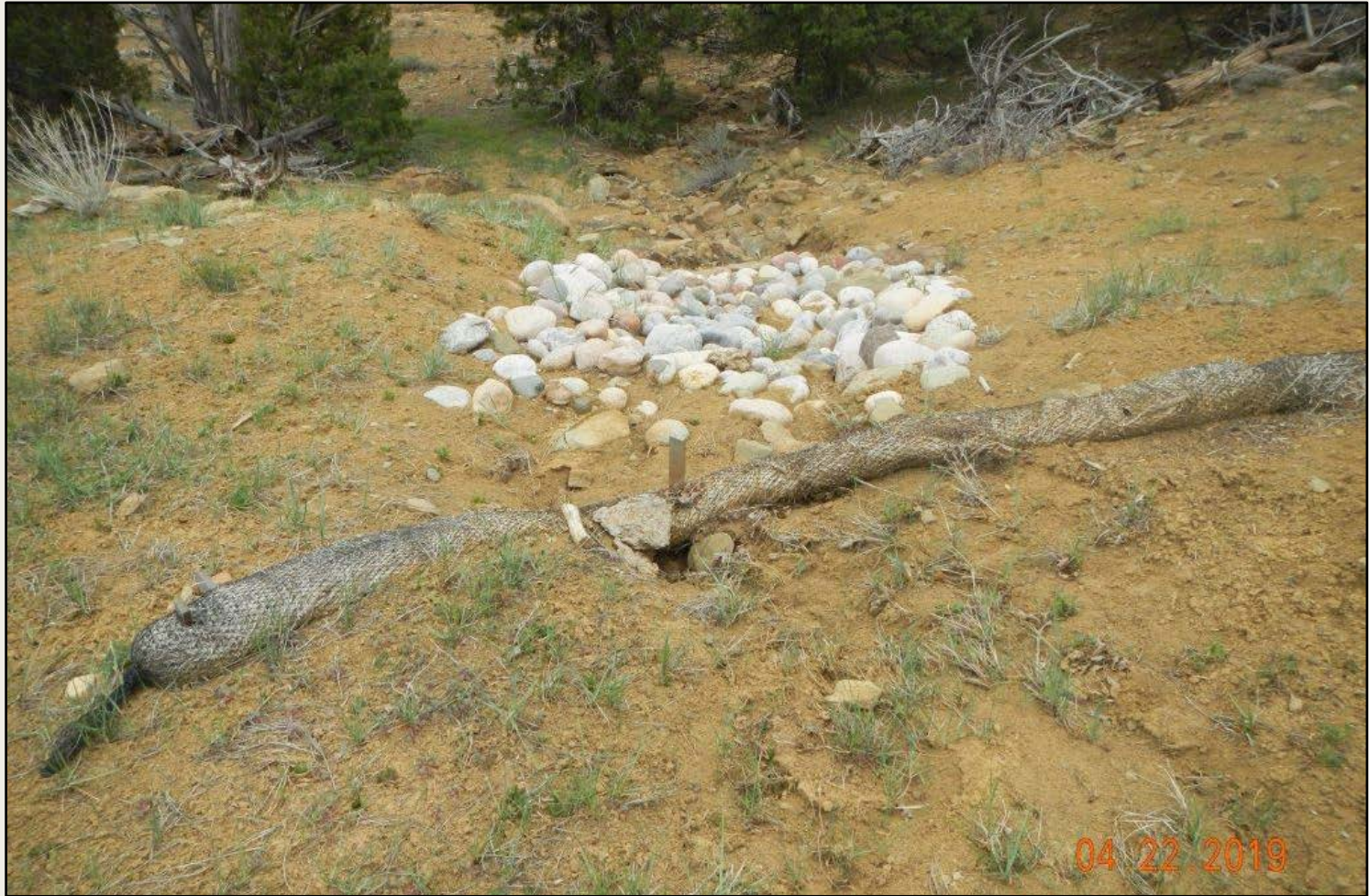
Photo 2. View of wattles and sediment deposition within the southeastern project area. Stormwater controls are not sufficient in this area.
