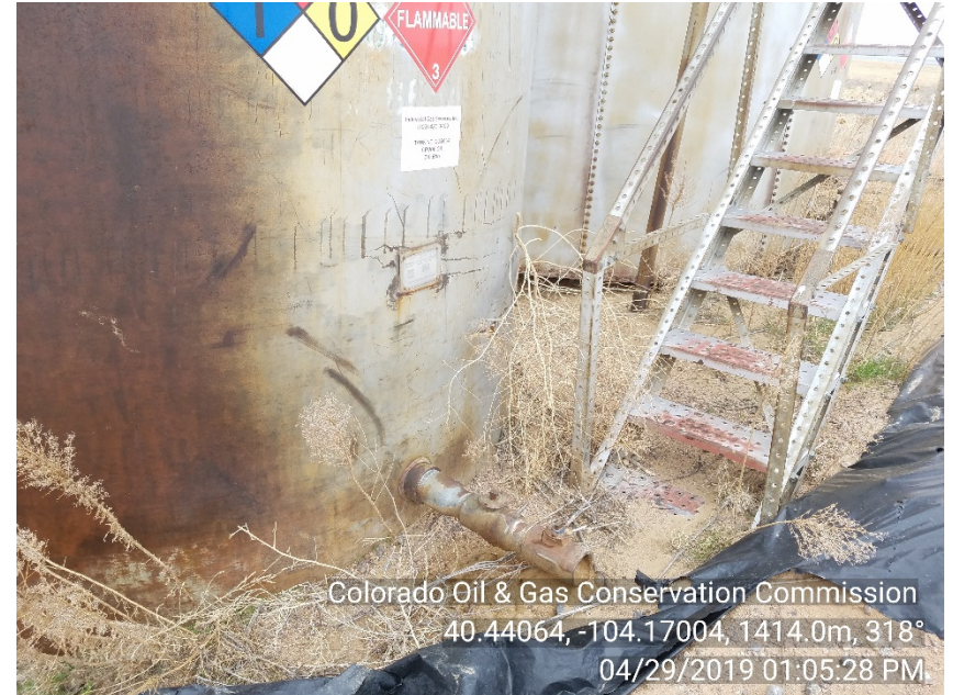
Photo #12 Behring #1 Crude oil tanks - Loadout Stained soil
