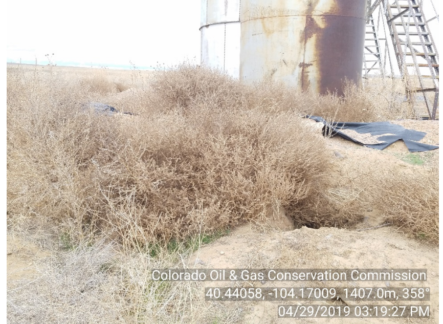
Photo #18 Behring #1 Crude Oil tanks Berms – Burrows, Weeds
