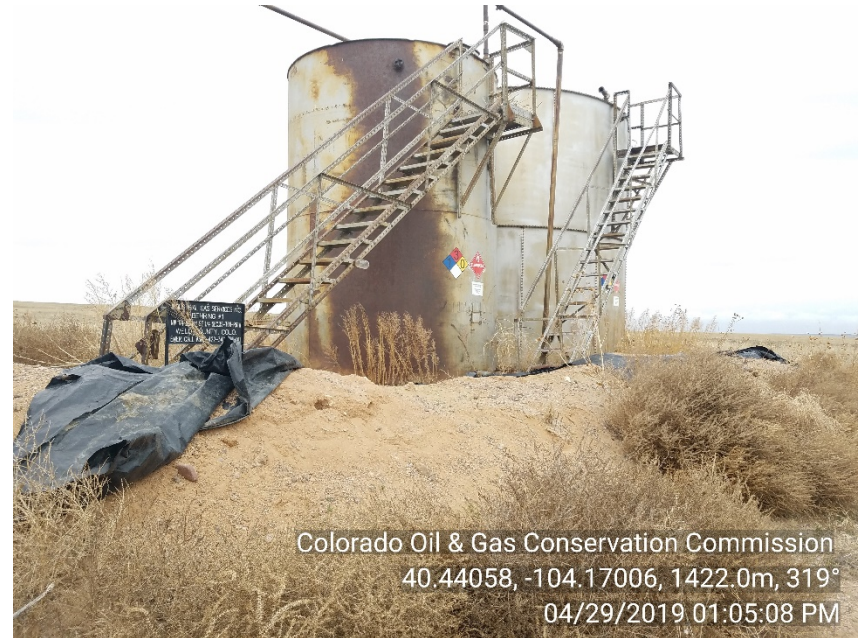
Photo #14 Behring #1 Crude oil tanks Rust
