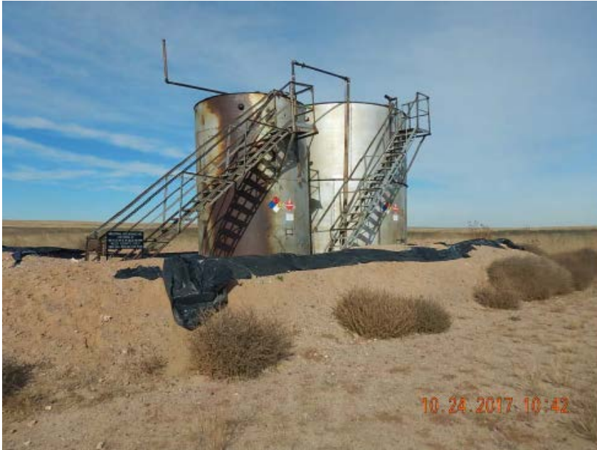
Photo #13 Behring #1 Crude oil tanks Rust from prior FIR
