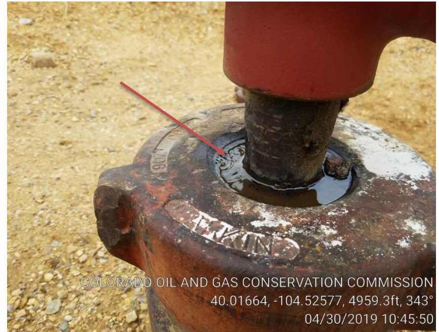
Pic 2 possible leak.
