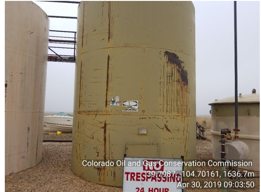
Photo 18 Labels and placards not litigable or not on crude oil tanks. Visual impact: tank visible from county road paint in disrepair.
