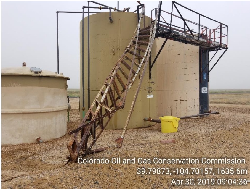
Photo 19 Unused equipment: Stairs in disrepair.
