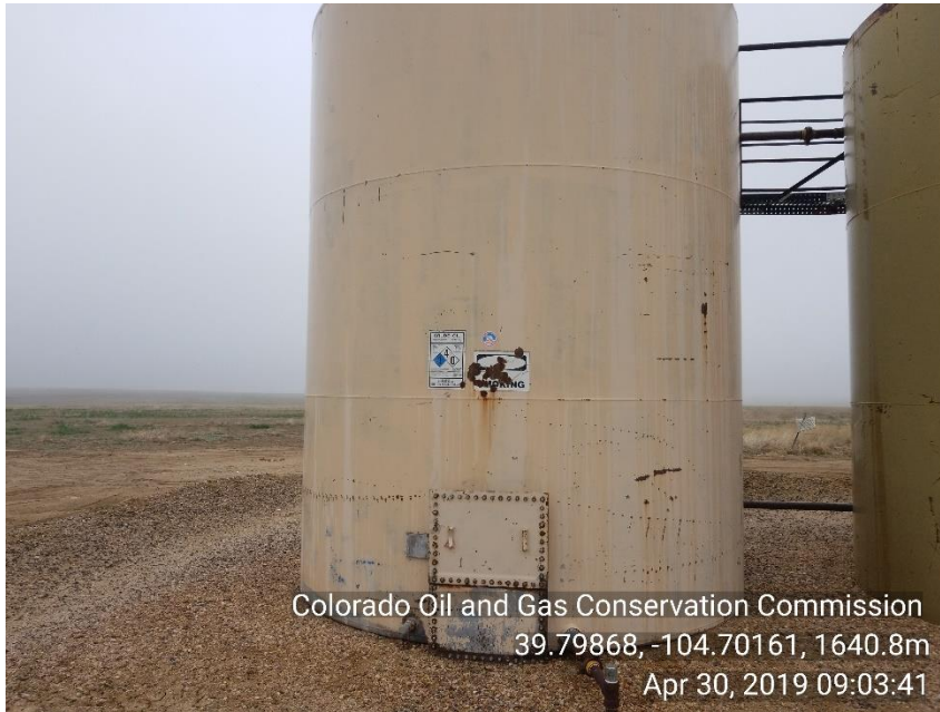
Photo 17 Labels and placards not litigable or not on crude oil tanks.
