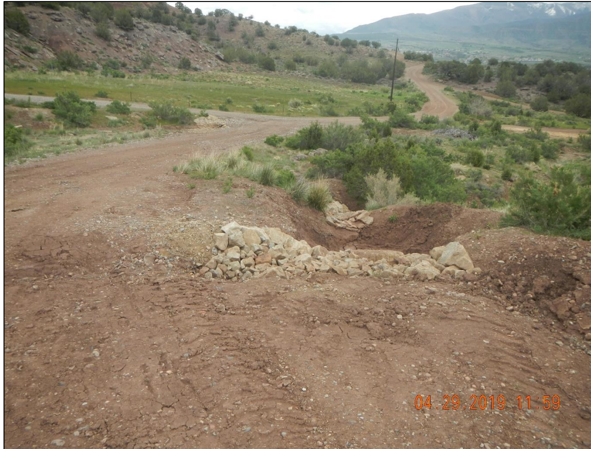
Checkdam repaired..
