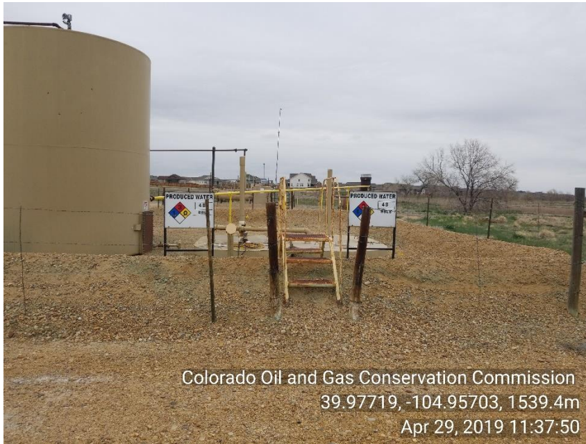
Photo 5 TNK BTRY. Production tanks Location located in a flood plain equipment not properly anchored and inadequate berm.
