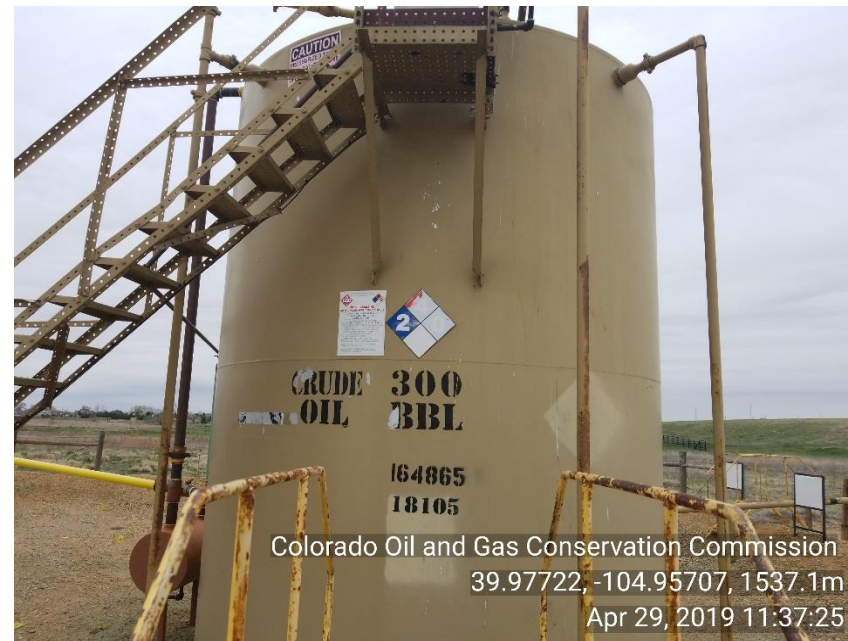
Photo 4 NFPA placard faded and illegible.
