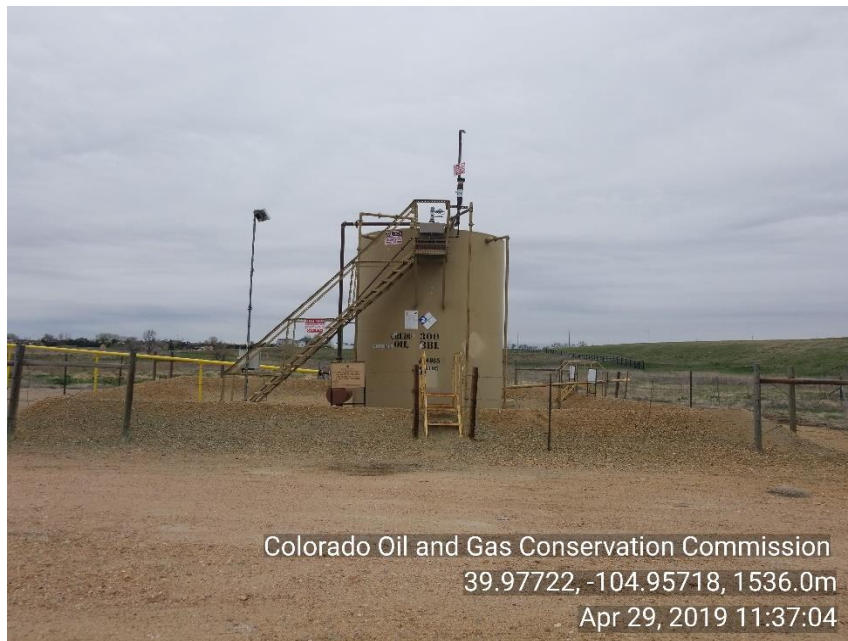
Photo 3 TNK BTRY. Location located in a flood plain equipment not properly anchored and inadequate berm.
