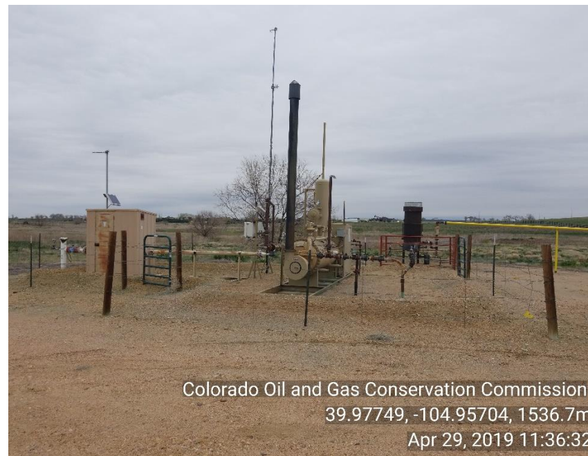
Photo 2 sep/meter house and ECD. Location located in a flood plain equipment not properly anchored and inadequate berm.
