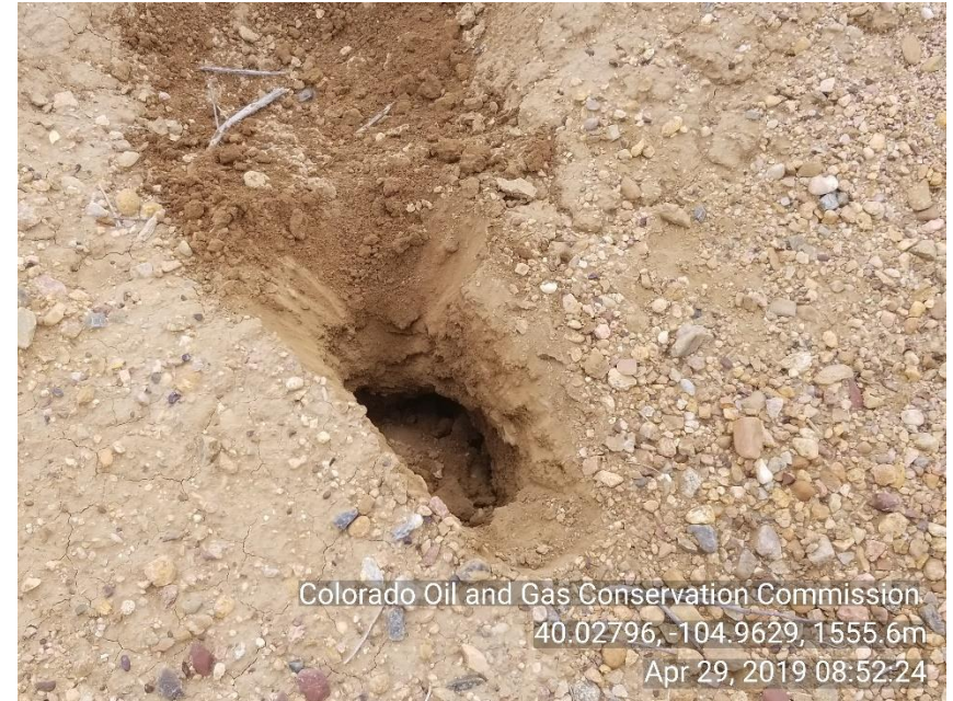
Photo 8 inadequate berm around crude oil tank. Burrows in containment walls.
