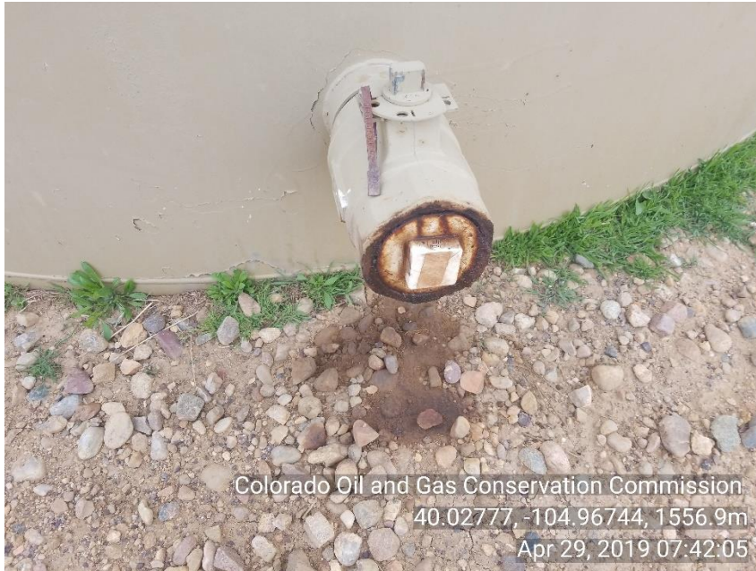
Photo 3 Stained soil under crude oil load out line. Mechanical issue Valve or bull plug appears to be leaking.
