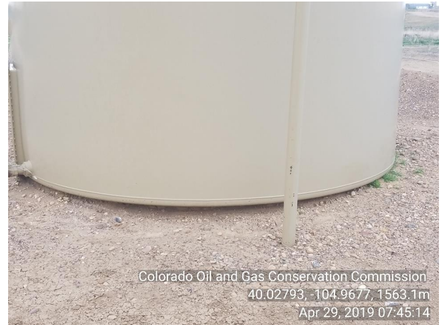
Photo 6 Crude oil tank gravel appears to be eroding away form underneath base of tank.
