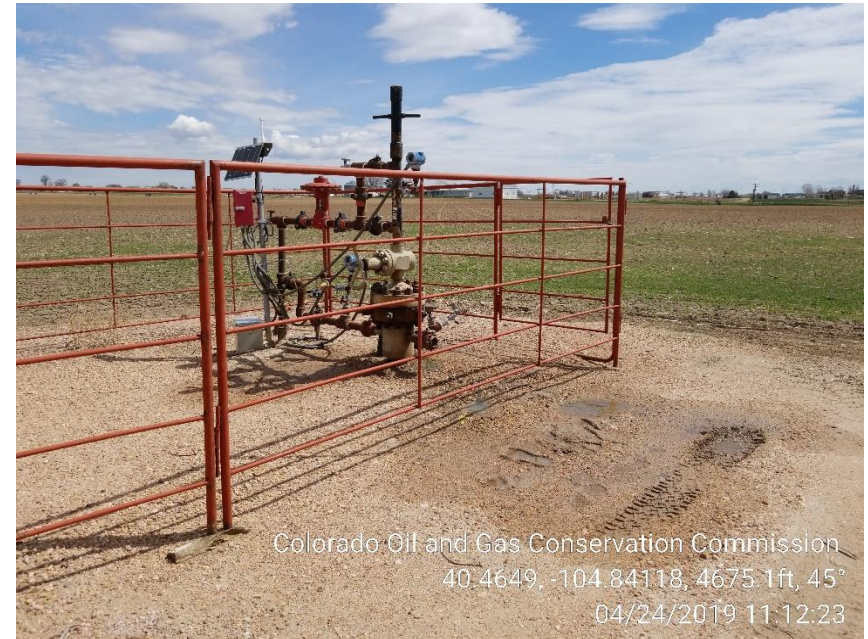
Photo 4 – Well Detterer FD 24-21D, API 123-35575, missing wellhead signage.
