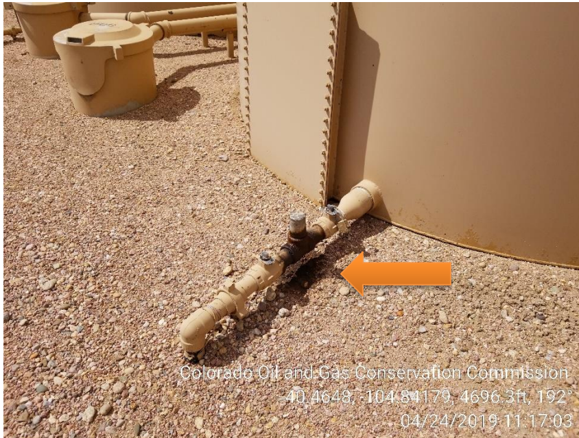
Photo 7 – Stained soil at the drain plug on the northeast Crude Oil tank.
