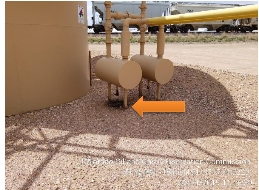
Photo 8 – Stained soil on south ECD knock-out pot, north side of Crude Oil tanks.
