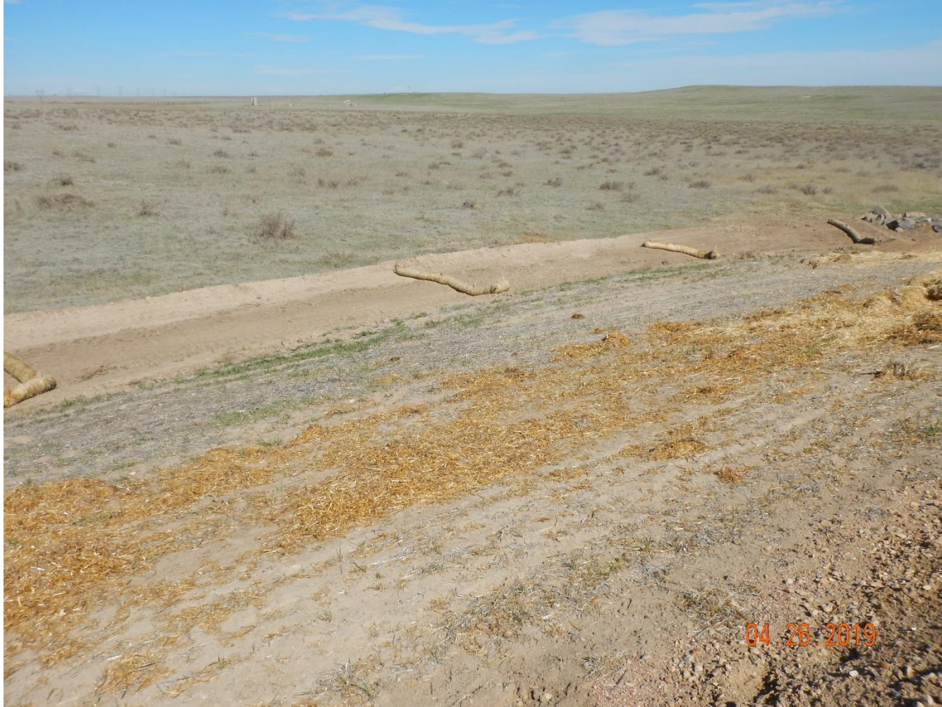
Photo 6: Photo taken from the northwest end of the location, facing northwest. Photo shows velocity checks within ditch.
