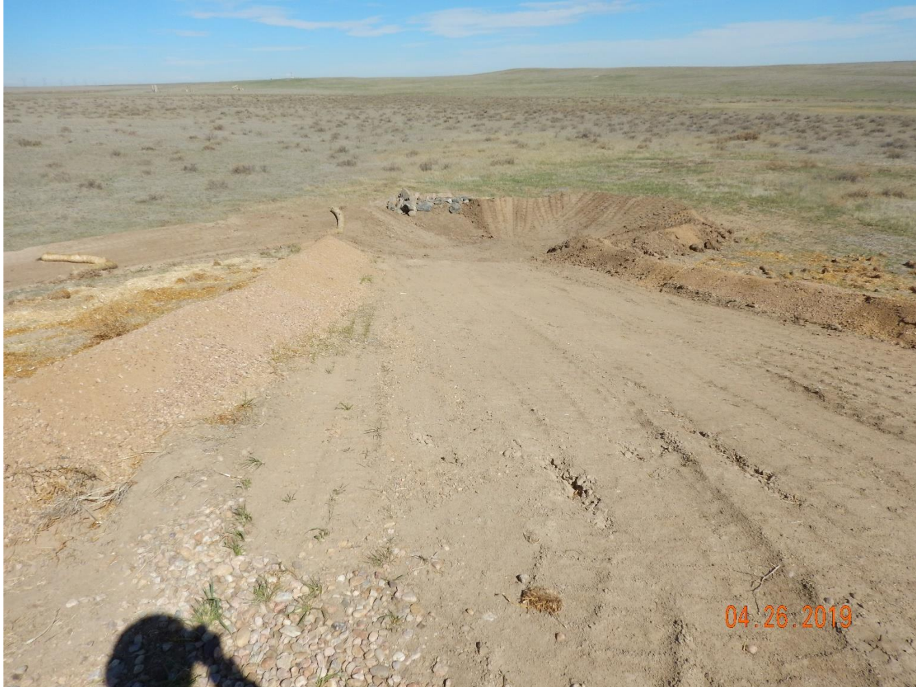
Photo 7: Photo taken from the northwest corner of the location, facing north. Photo shows operator has updated the sediment trap.
