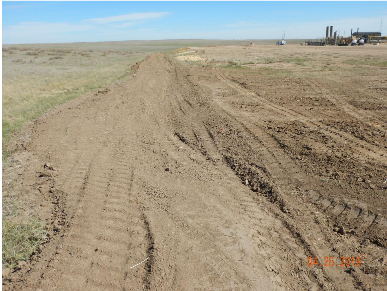
Photo 3: Photo taken from the southwest end of the pad, facing north. Photo shows operator has installed a stormwater ditch on the western perimeter of the pad.
