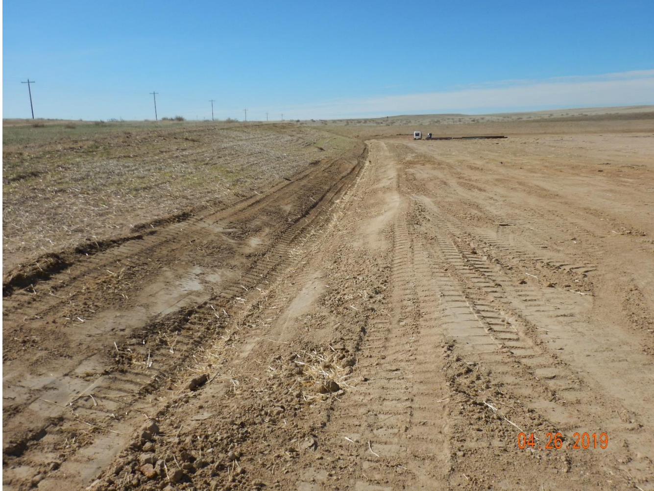
Photo 1: Photo taken from the east end of the location facing south. Photo shows operator has installed a ditch along the eastern perimeter of the pad.
