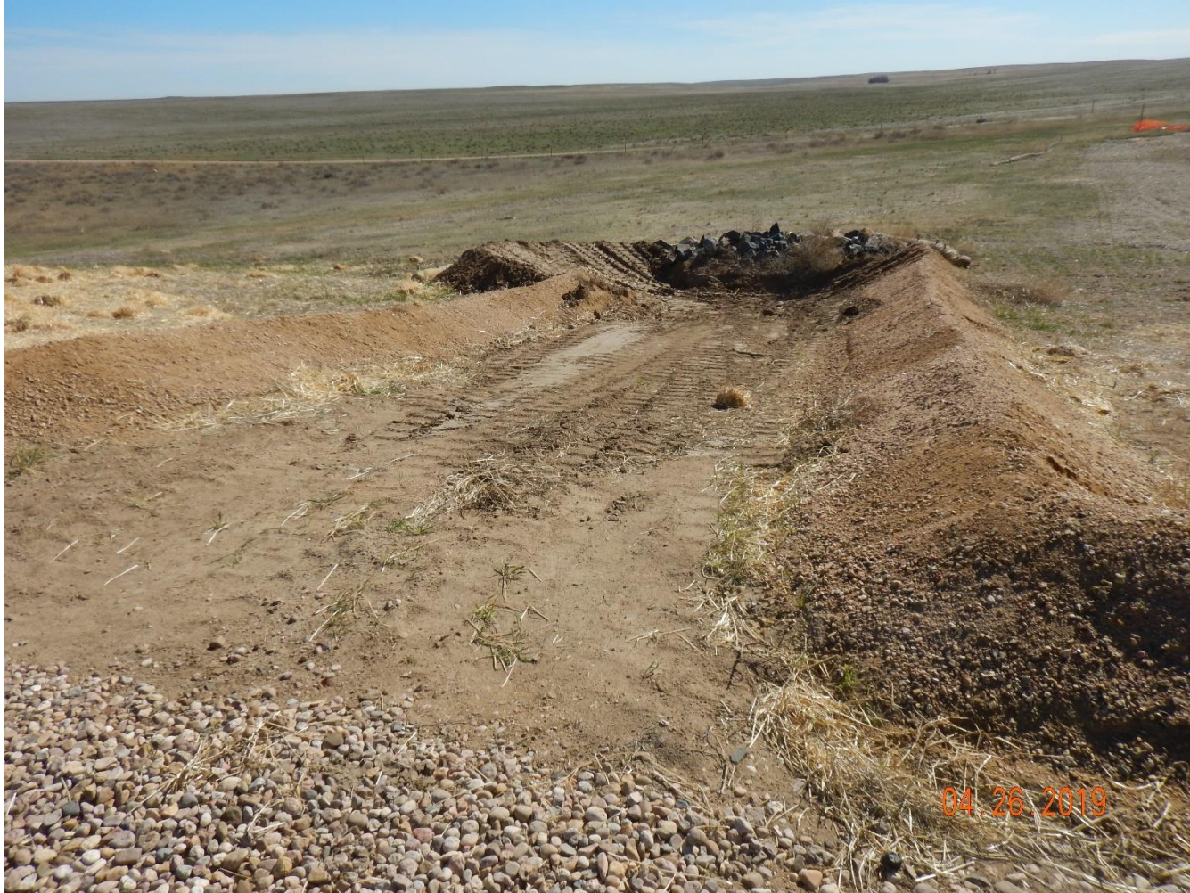
Photo 8: Photo taken from the northeast corner of the location, facing east. Photo shows operator has updated the sediment trap.
