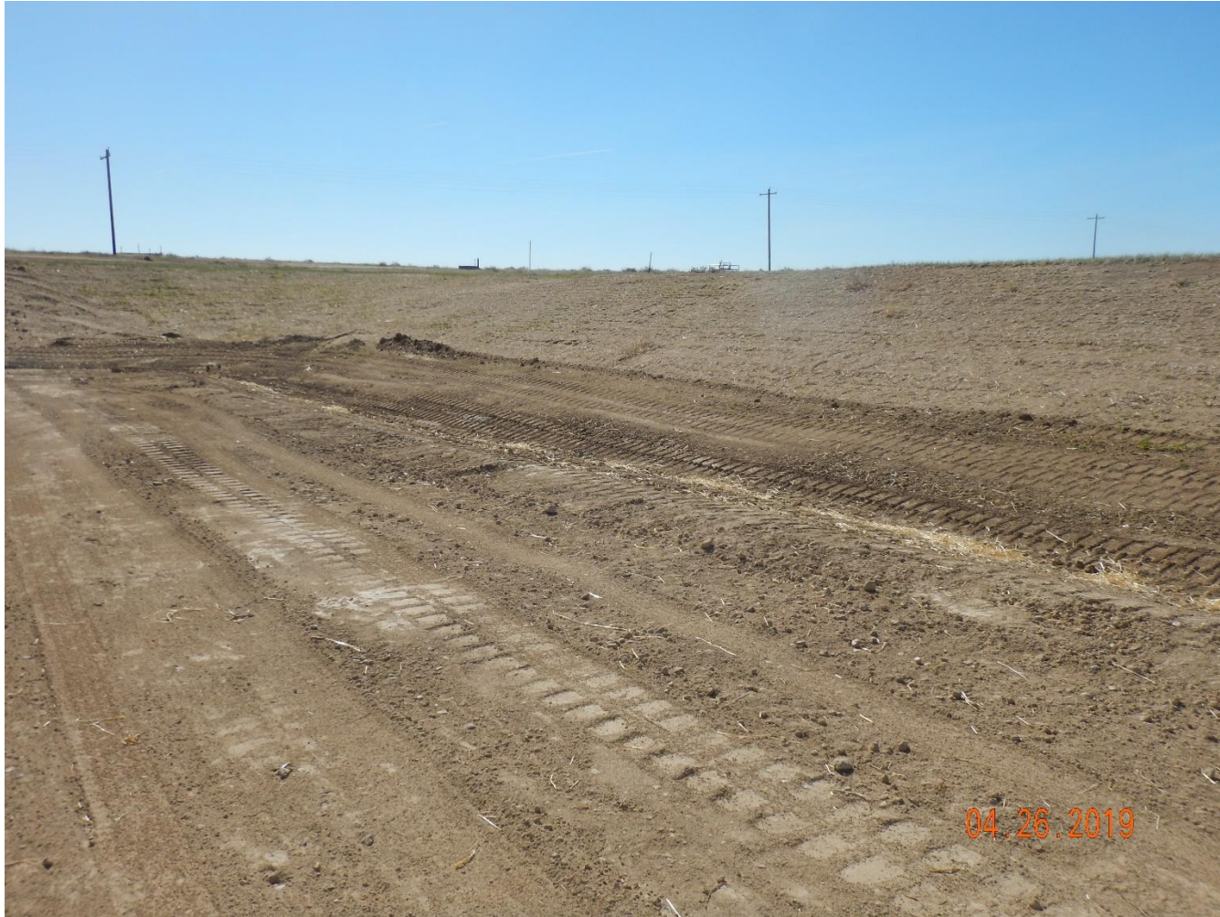
Photo 2: Photo taken from the southeast end of the location, facing southeast. Photo shows operator has installed a ditch. Photo also shows erosion degradation has been repaired and slopes appear to have been seeded/mulched.
