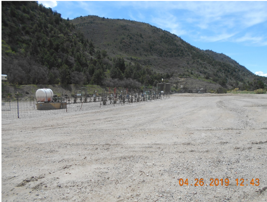
Overview of location looking SW.
