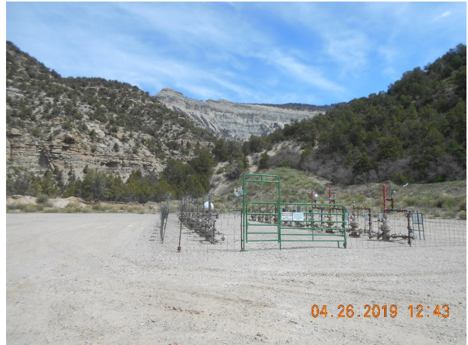
Wellheads with fencing
