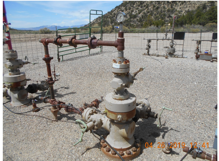
Injection wellhead
