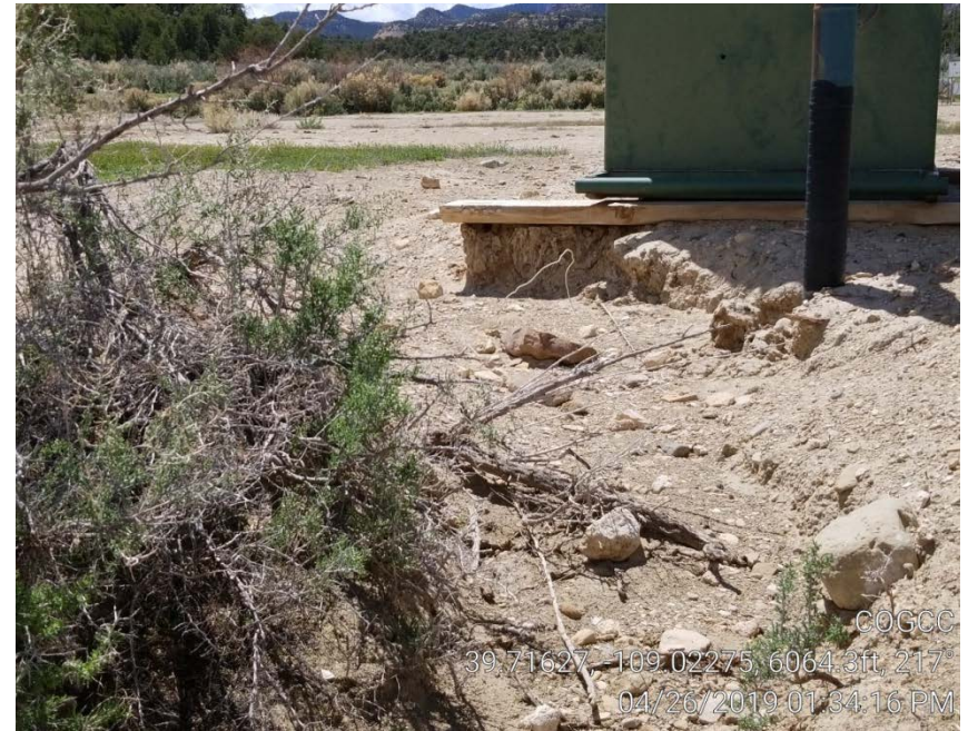
Photo 2. Erosion channel next to separator from storm water leaving location.
