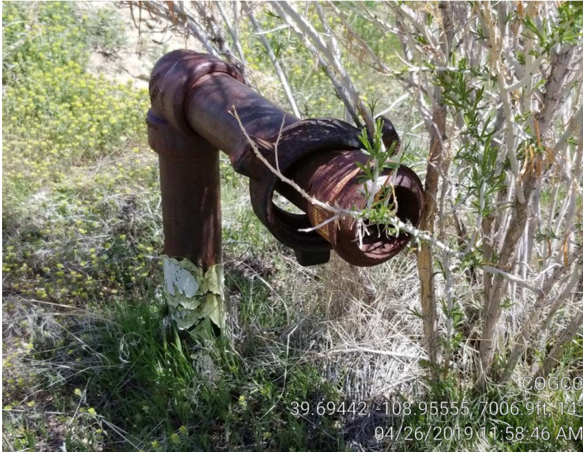
Photo 3. Uncapped riser between meter building and pit.
