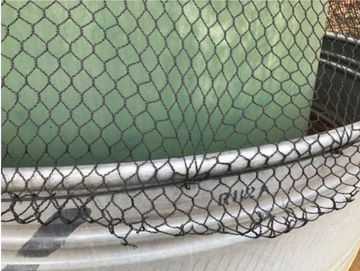
PHOTO 3: THE NETTING COVERING THE TANK WAS REPAIRED AND REFASTENED TO SECURE NET TO TANK.
