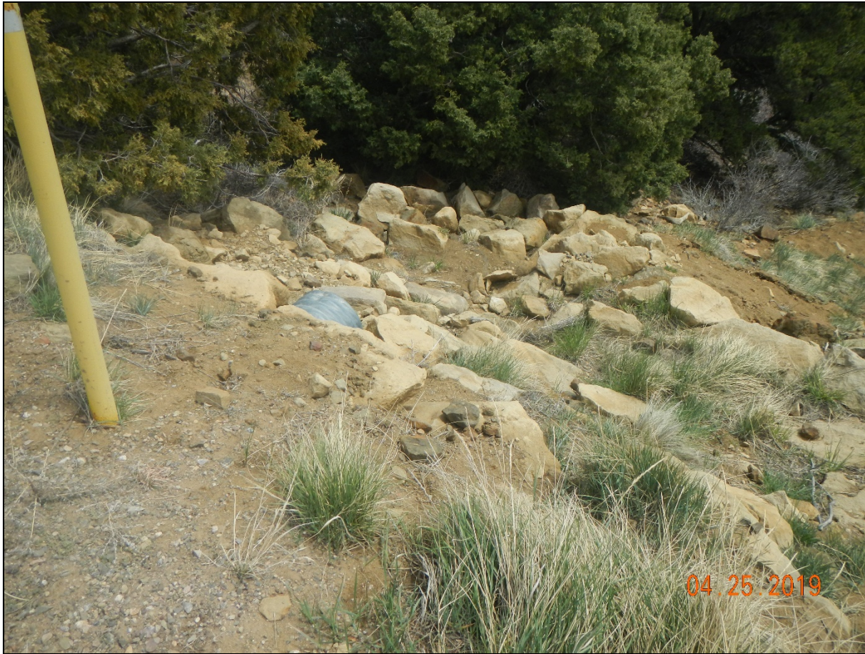
Photo 4. Culverts appear to be properly installed and maintained.
