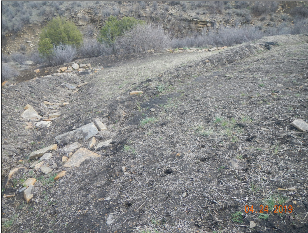
Photo 2. Facing off the north fill slope. Berms and rock rip/rap are installed for stormwater control.
