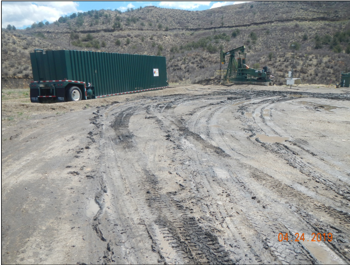
Photo 1. Facing toward the wellhead. There is some vehicle rutting this area may need more gravel.
