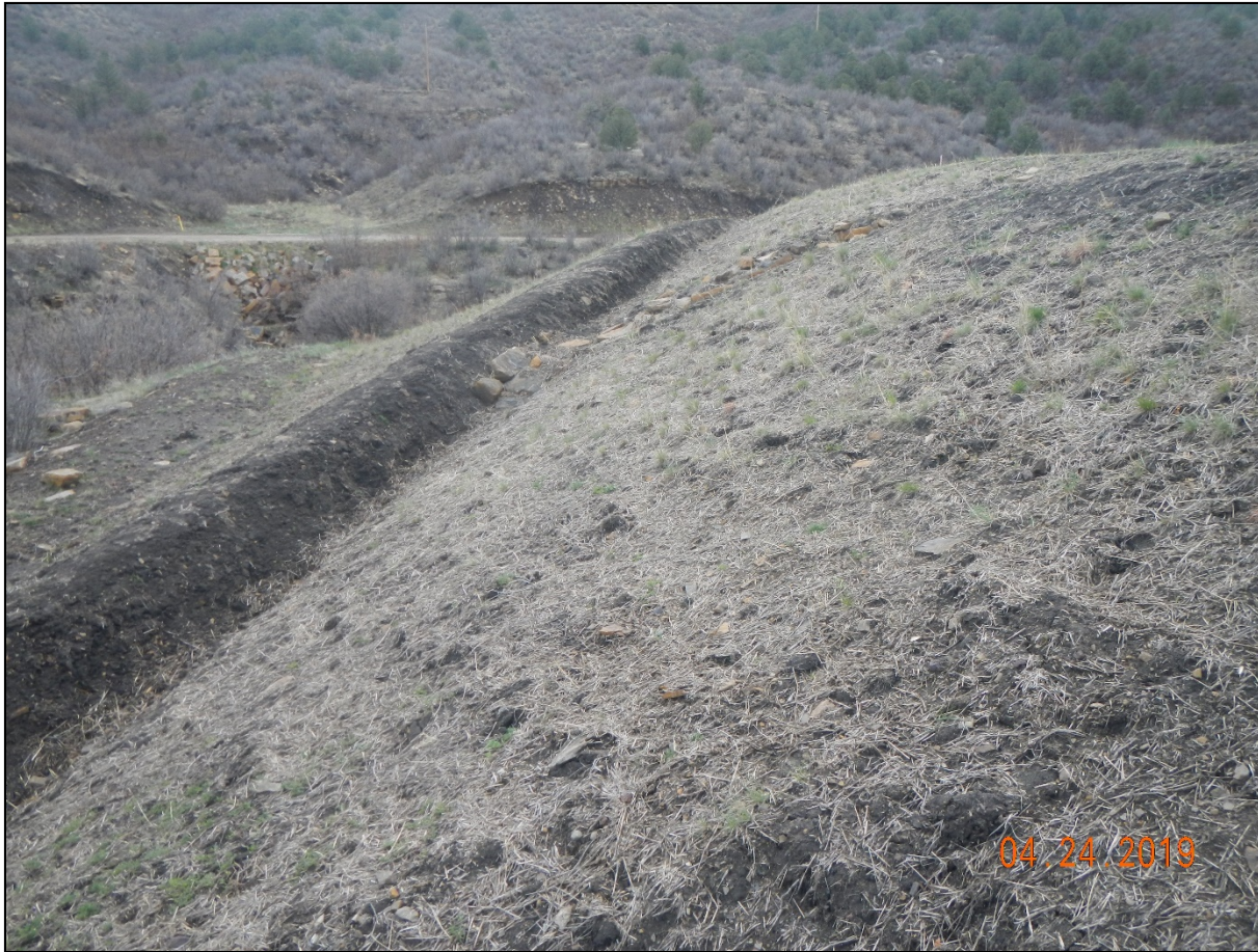
Photo 3. The fill slope was mulched and seeded. Vegetation is beginning to establish.
