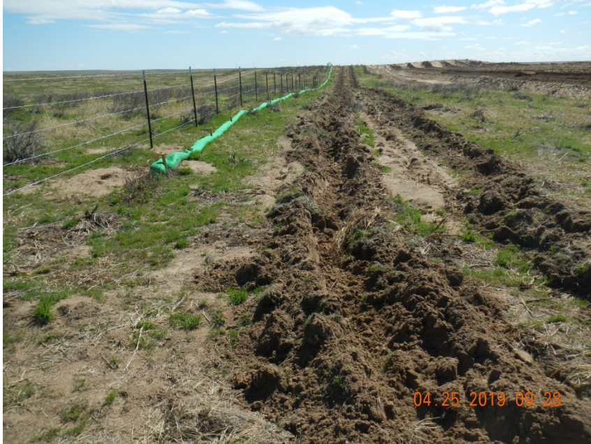
Photo 3. Photo taken from the northern perimeter of the location, facing East. Appears the Operator has installed filtrex BMPs around the perimeter of the location.
