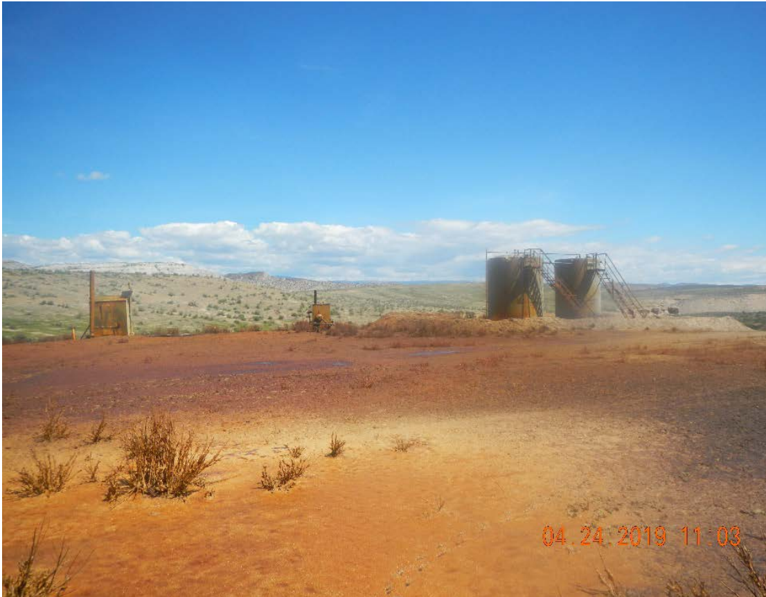
Photo 3-Looking north. Note pooling of oil on access road in truck ruts.
