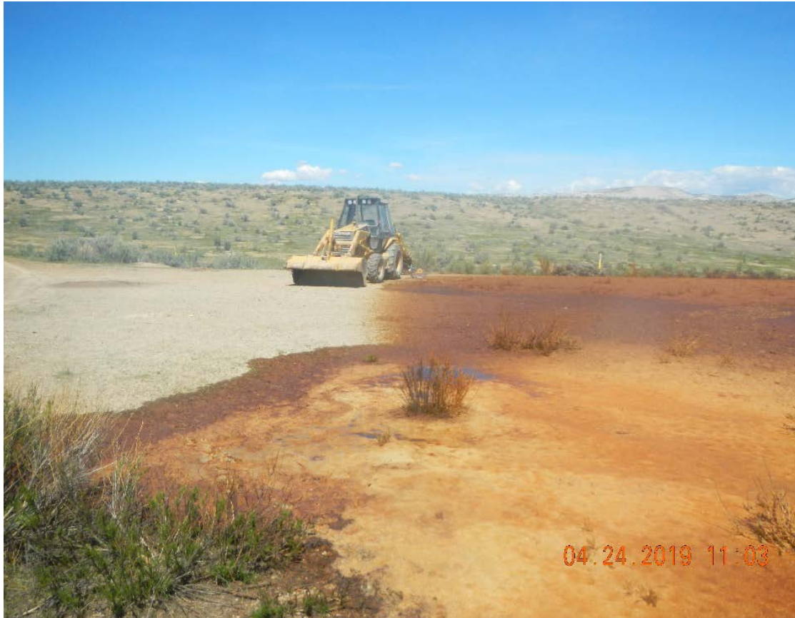
Photo 2-Wellhead is behind and to the left of camera, looking north . Note: treater in right center at the edge of pad for reference. Note pooling of oil in truck ruts.
