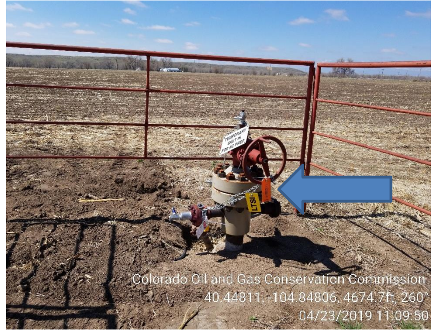
Photo 2 – Wellhead now has the Orange Decommission tag installed
