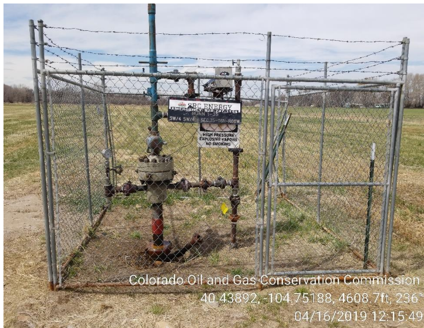
Photo 1 – Wellhead, unused equipment has been removed from location.
