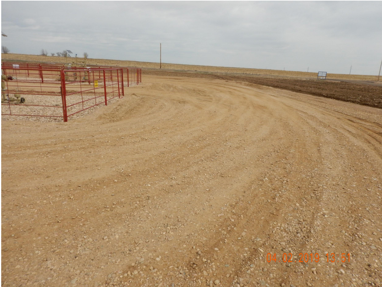
Photo 2. Photo taken from the southwestern well location, facing East. A gravelled berm BMP has been installed around the perimeter of the location.
