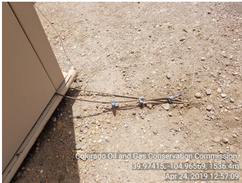
Photo 5 Separator anchoring
