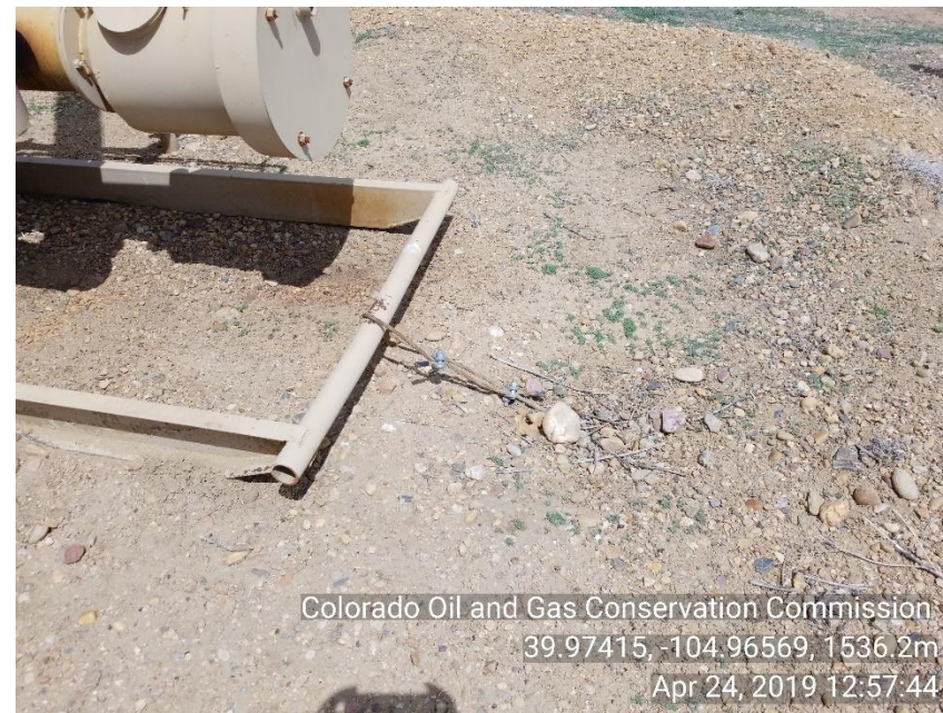
Photo 6 Separator anchoring
