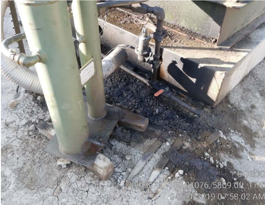
Photo 5. Oily soil near pump jack motor.
