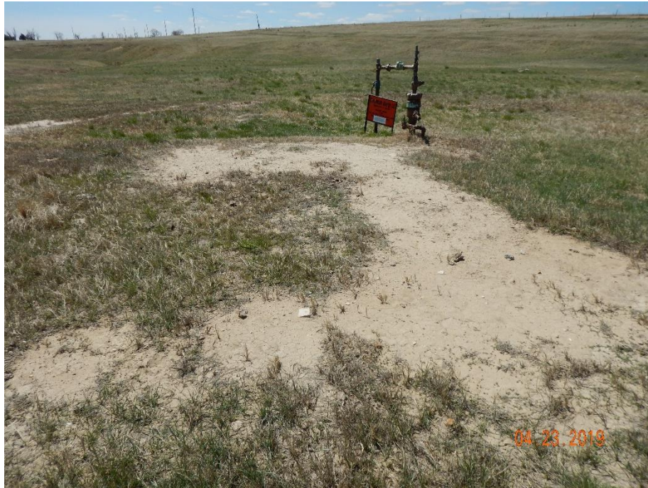
Photo 1: Photo taken from the north end of the location, facing south. Photo shows undesirable weedy plant species such as kochia and salsola sp. have established on areas adjacent to well head.
