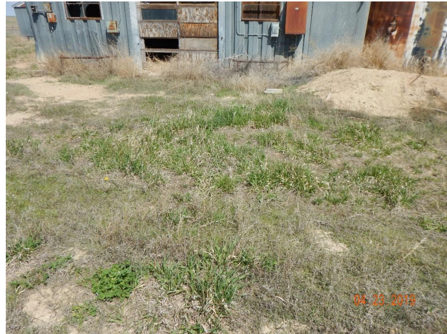
Photo 8: Photo shows undesirable weedy plant establishment, and weed debris accumulation on berms and equipment.
