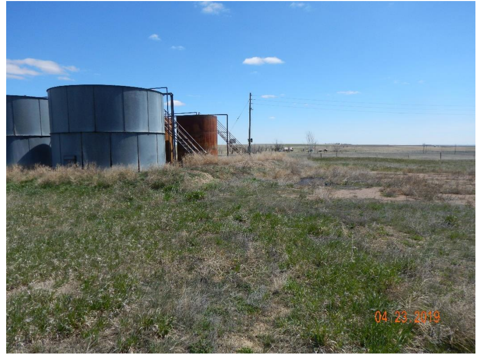
Photo 2: Photo taken from the southwest end of the tank battery, facing east. Photo shows weed debris accumulation on the berms and around equipment.
