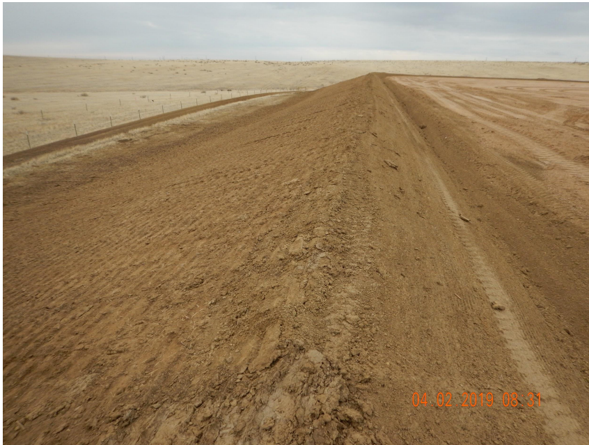
Photo 1. Photo taken from the eastern well location, facing South. Photo illustrates a ditch installed around the perimeter of the well pad which will be directed to a sediment trap. The eastern fill slope has been temporarily stabilized with equipment tracking.
