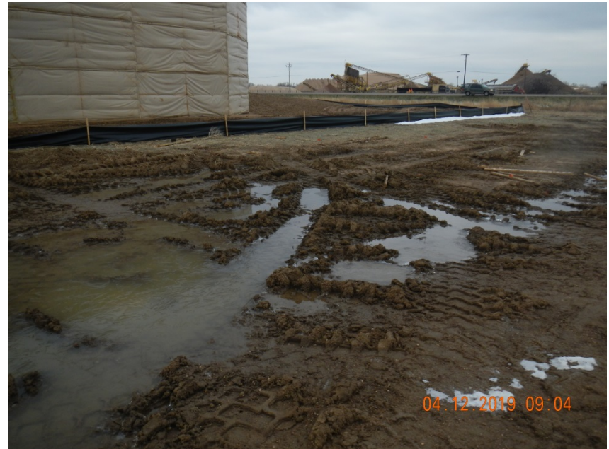
Photo 6. Photo taken from the northwestern perimeter of the location, facing East. Photo depicts the silt fence BMP that has been installed.
