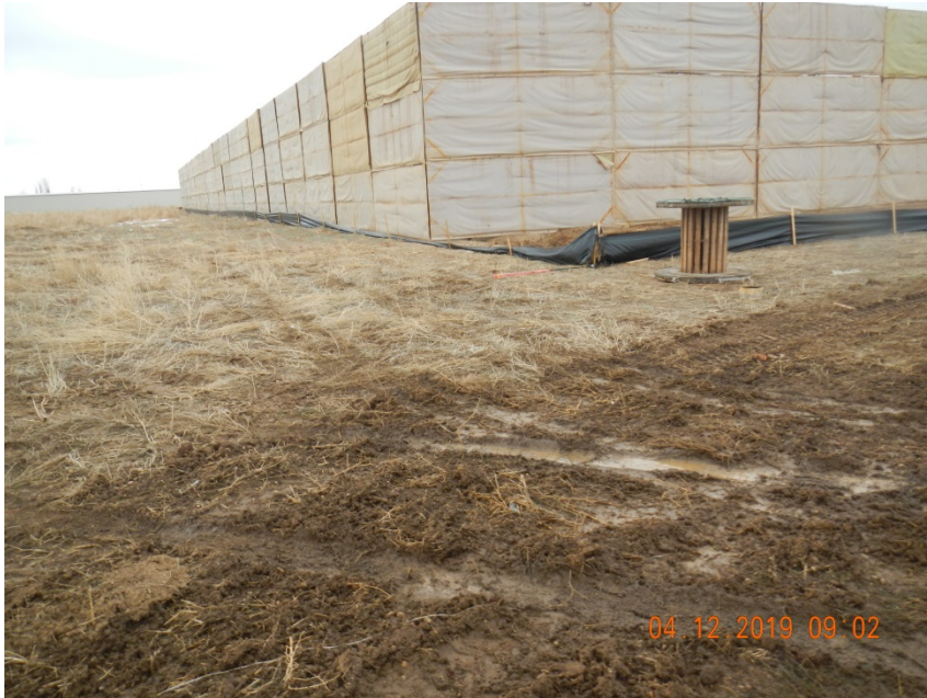
Photo 3. Photo taken from the northeastern perimeter of the location, facing South. Photo illustrates the installed silt fence BMP is not in proper functioning condition.
