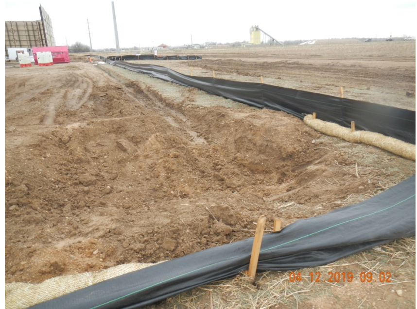
Photo 4. Photo taken from the northwestern perimeter of the location, facing East. Photo illustrates a sediment trap installed however no stabilized outlet is apparent.
