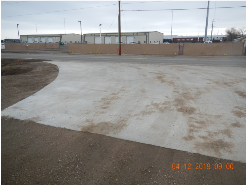
Photo 1. Photo taken from the entrance to the access road Off CR 27, facing Northeast. Photo illustrates a concrete pad installed by the Operator to potentially limit tracking on to the county road.
