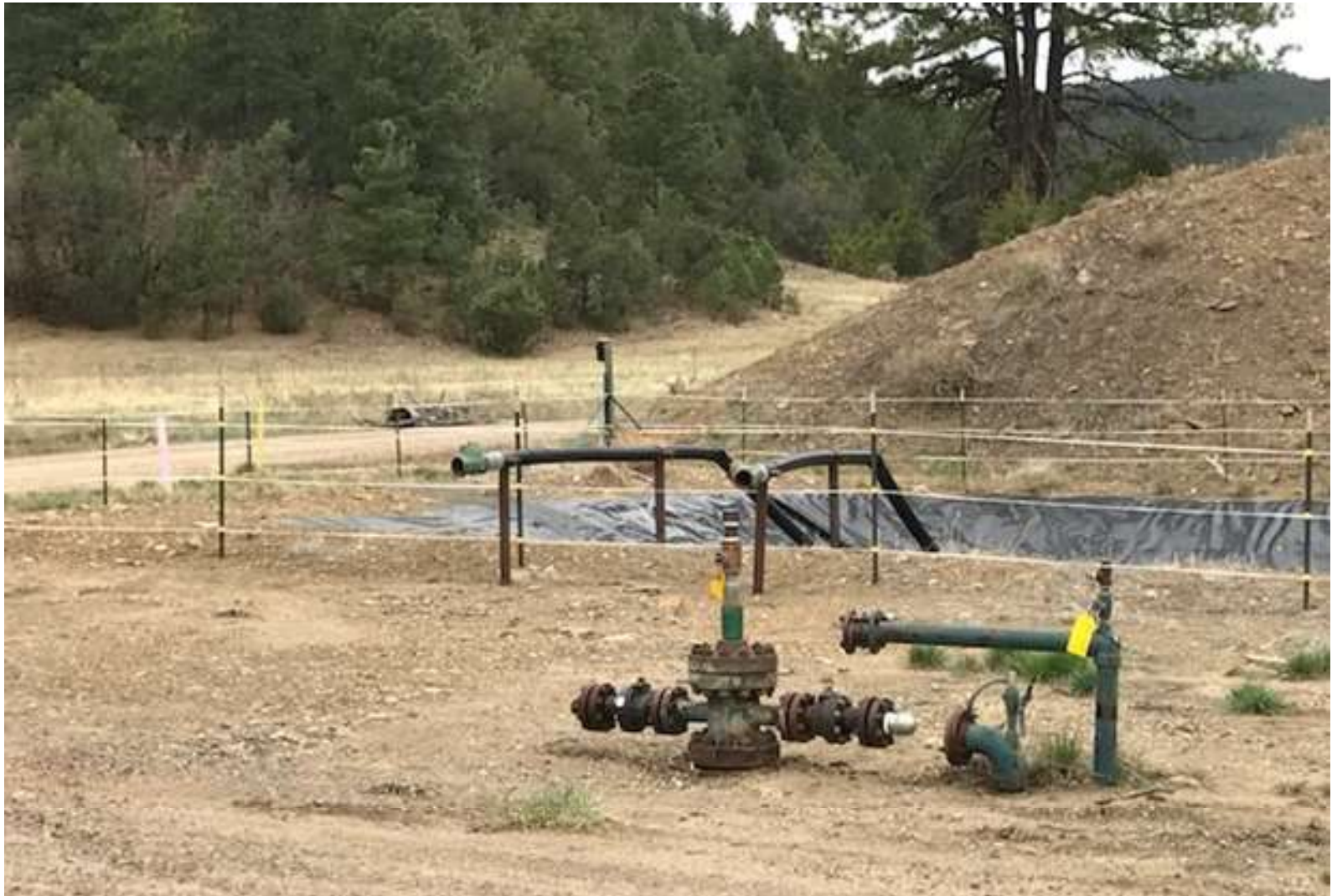
PHOTO 5: THE FENCE SURROUNDING THE PRODUCTION PIT HAS BEEN REPAIRED.
