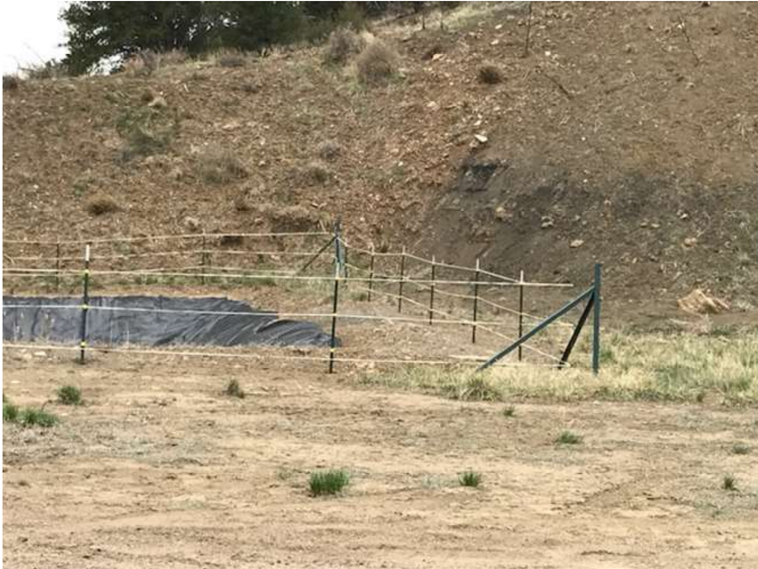
PHOTO 4: THE FENCE SURROUNDING THE PRODUCTION PIT HAS BEEN REPAIRED.
