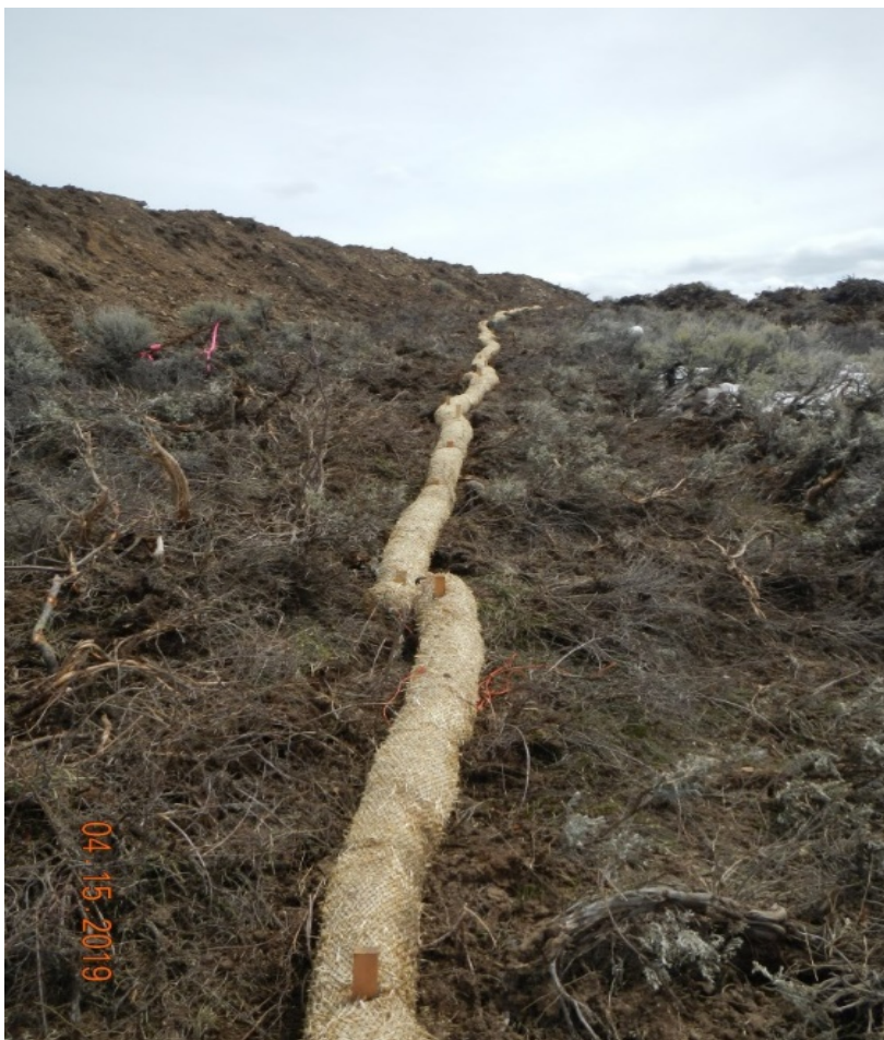
Photo#7: Wattles have been installed as Perimeter control.
