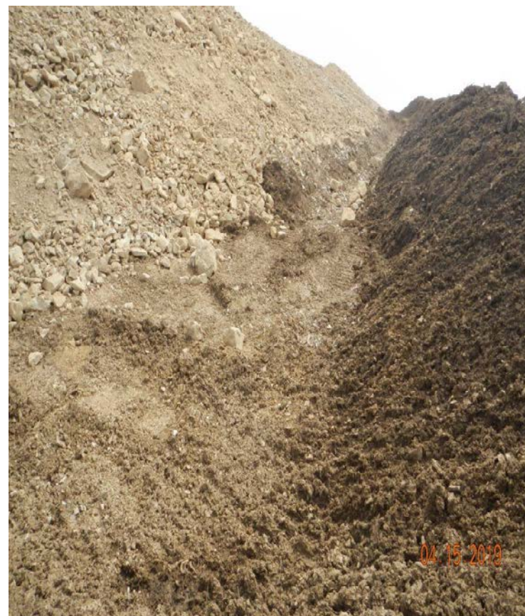
Photo#6: Topsoil windrowed along toe of Fill slope
