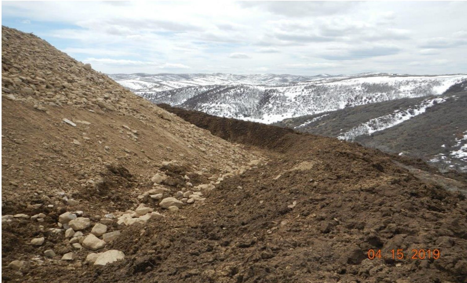
Photo#4: Topsoil windrowed along toe of Fill slope
