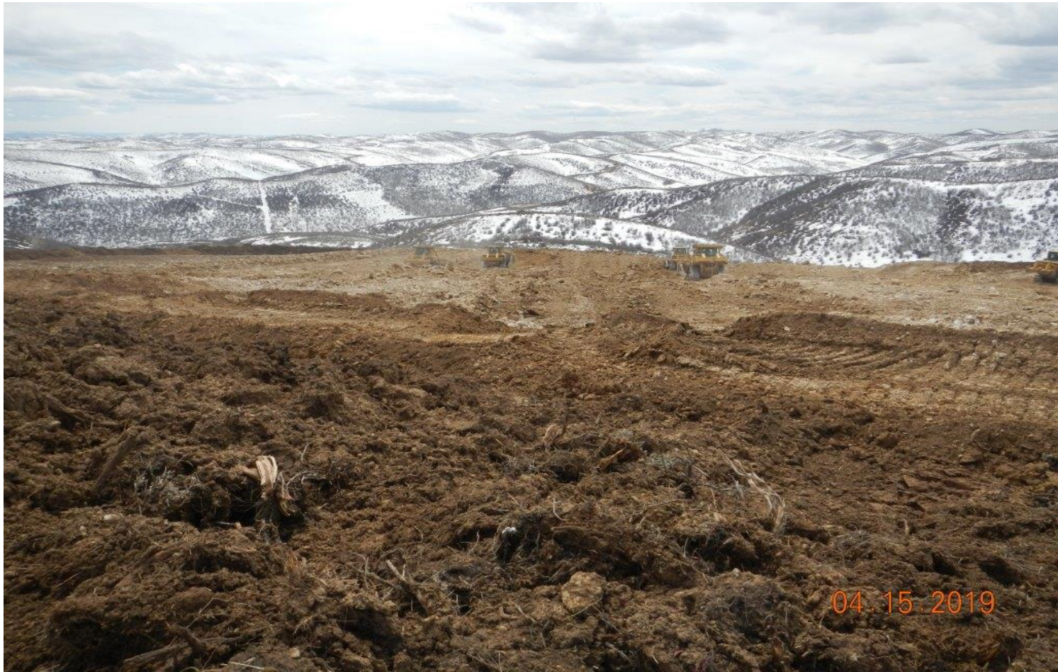
Photo#1: Overview of Location from top of Cut slope to Southwest.
