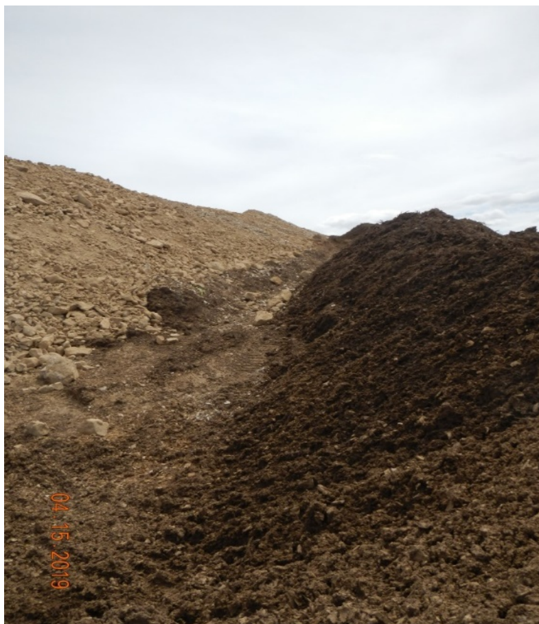
Photo#5: Topsoil windrowed along toe of Fill slope
