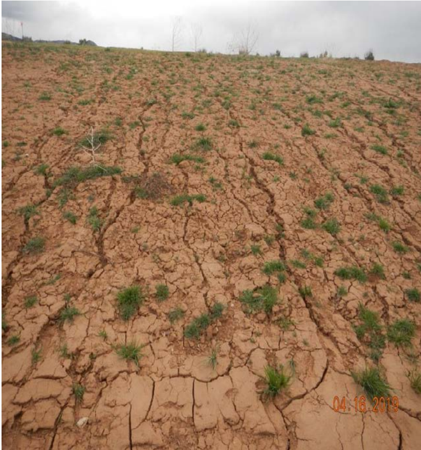
Photo#8: Erosion concerns on cut slope.
