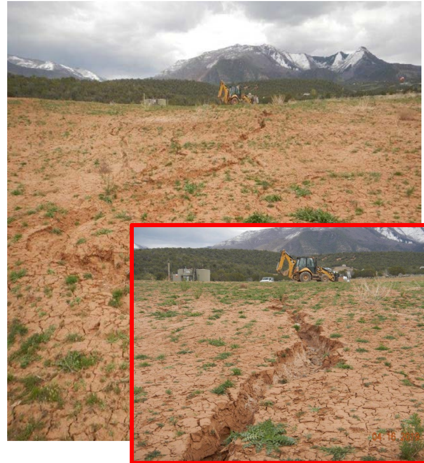
Photo#5: Stormwater cutting channels, washing out vegetation.
