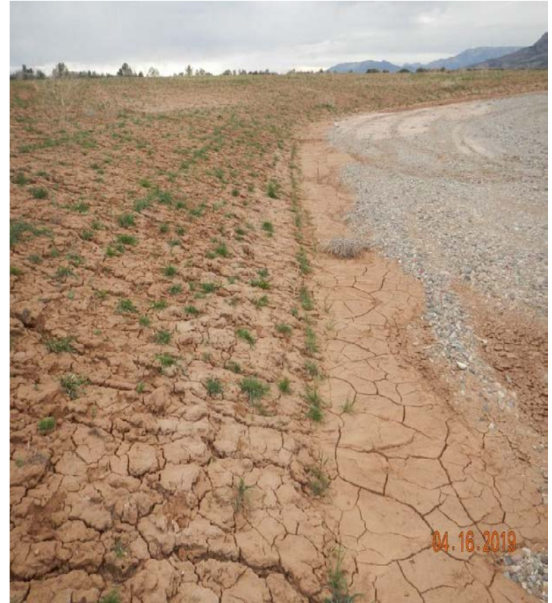
Photo#9: Erosion concerns on cut slope.
