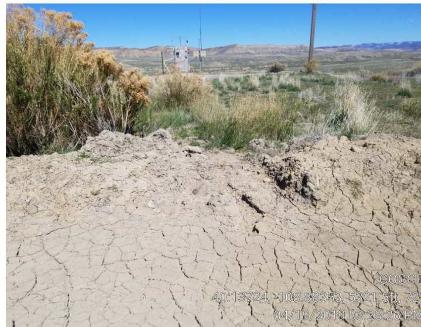
Photo 2. Stormwater berm breach on east edge of location.
