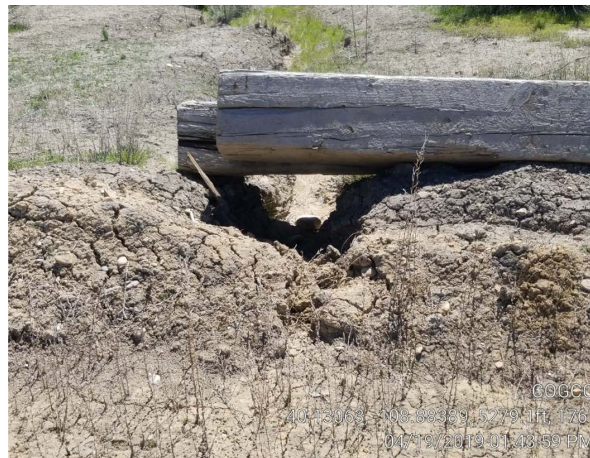
Photo 2. Stormwater berm breach on south edge of location.
