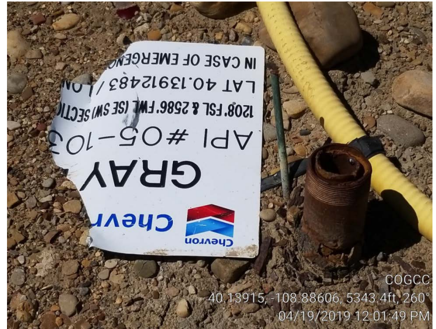
Photo 2. Unused sign & uncapped riser.
