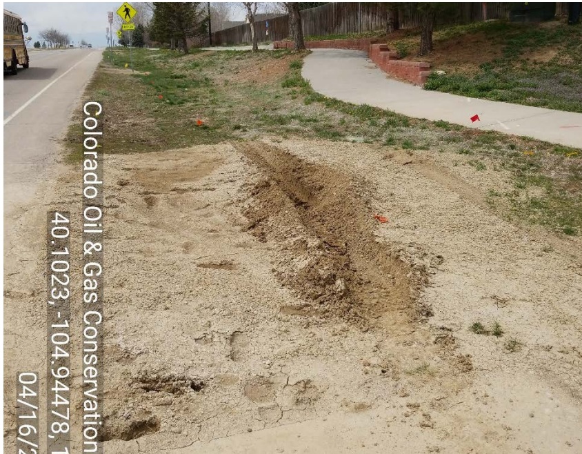
Reclaimed excavation to expose damaged section of a flowline. Excavation was opened on 03/28/2019. Tipple Parkway is visible to the left of the excavation.
