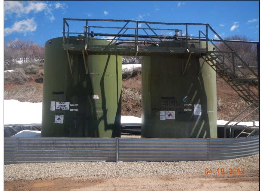
Photo of tank battery
