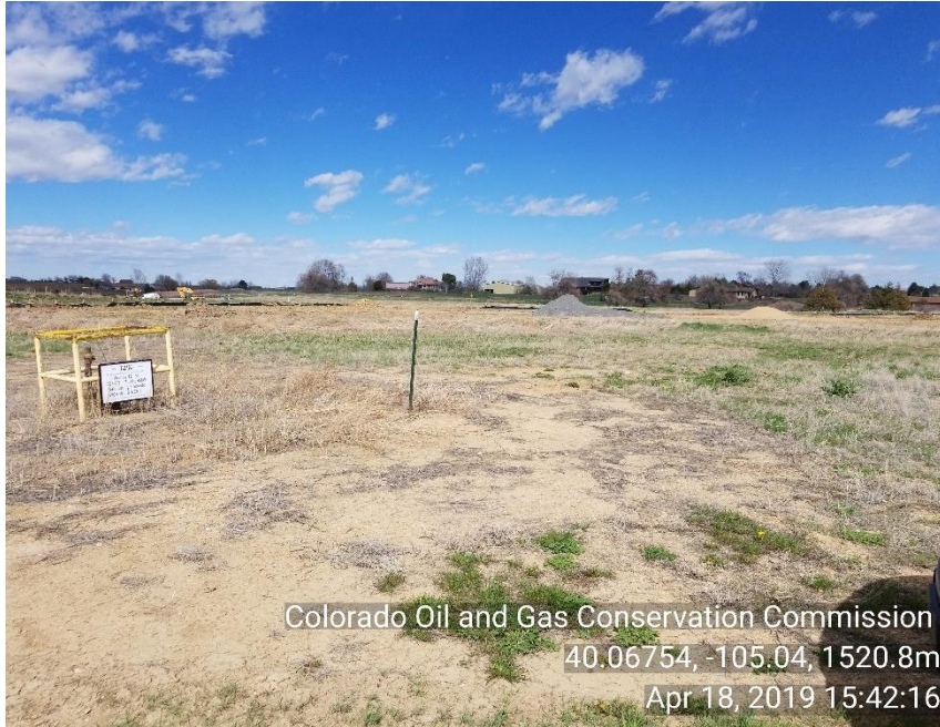
Photo 1 Well is P&A other well on site is KPK
