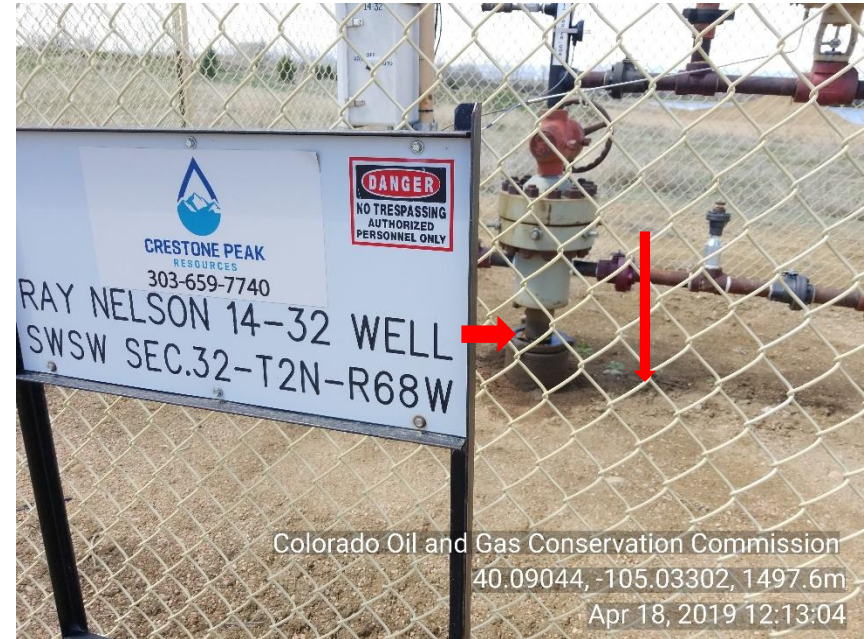
Photo 6 Ray Nelson #14-32 Stained soil around well head. Mechanical issue appears well head is leaking.
