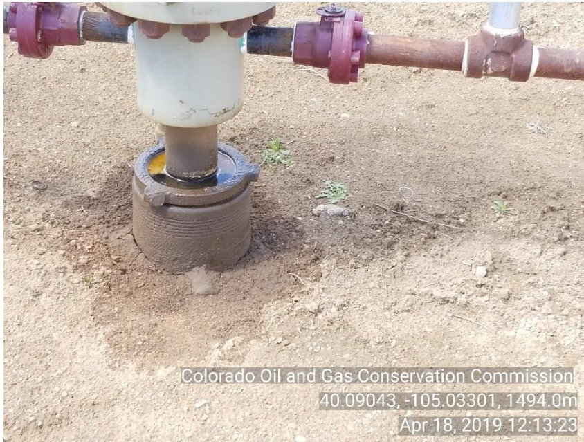
Photo 7 Ray Nelson #14-32 Stained soil around well head. Mechanical issue appears well head is leaking.
