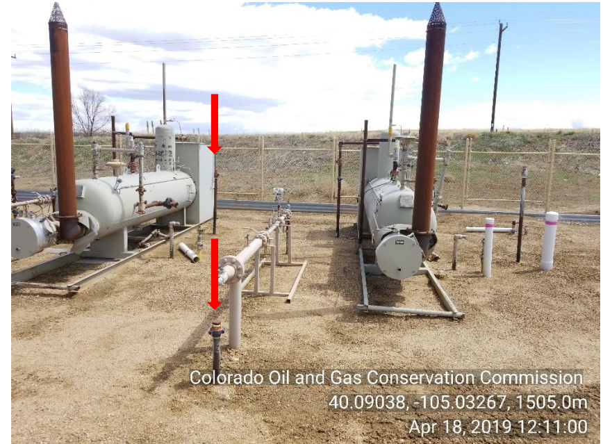
Photo 4 Unused equipment (separators 2) Unmarked unused and not LOTO risers
