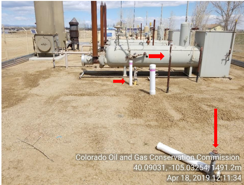
Photo 5 Unused equipment (separators 2) Unmarked unused and not LOTO risers
