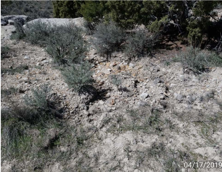
Photo 3. Run off from the northwest side of the location through a breached berm.
