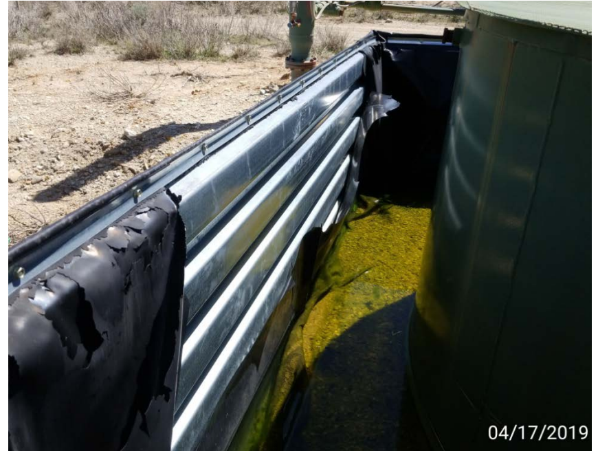
Photo 2. Tank liner is torn.
