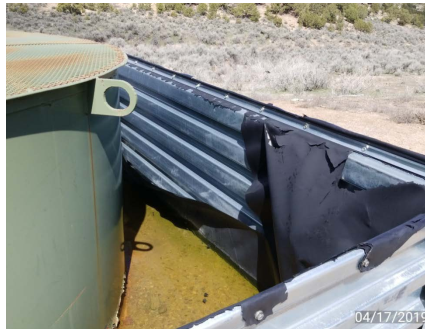
Photo 2. Tank liner is torn.
