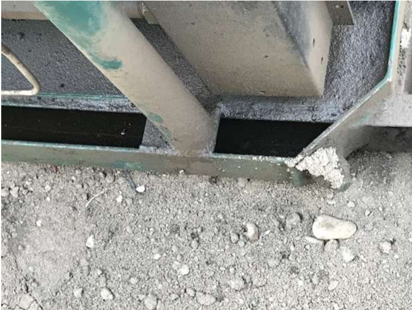
PHOTO 1: THE ACCUMULATED OIL WAS REMOVED FROM THE COMPRESSOR'S RESERVOIR.
