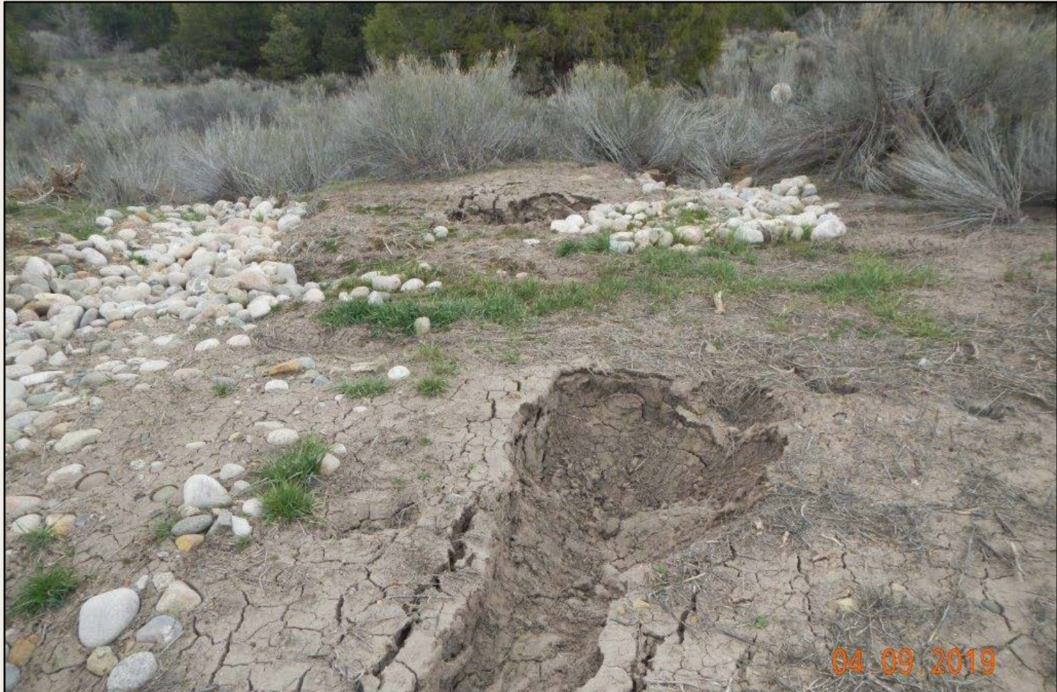
Photo 4. View of erosional tunneling within the eastern project area. Cobble BMP is not and adequate sto
