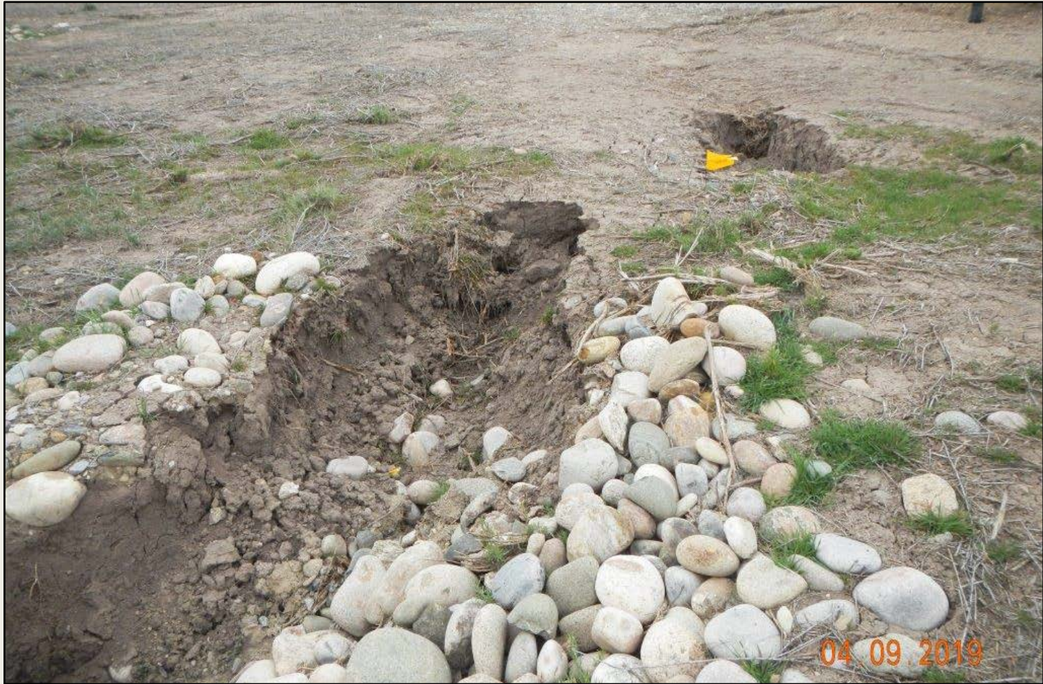
Photo 5. View of more erosional tunneling within the eastern project area.
