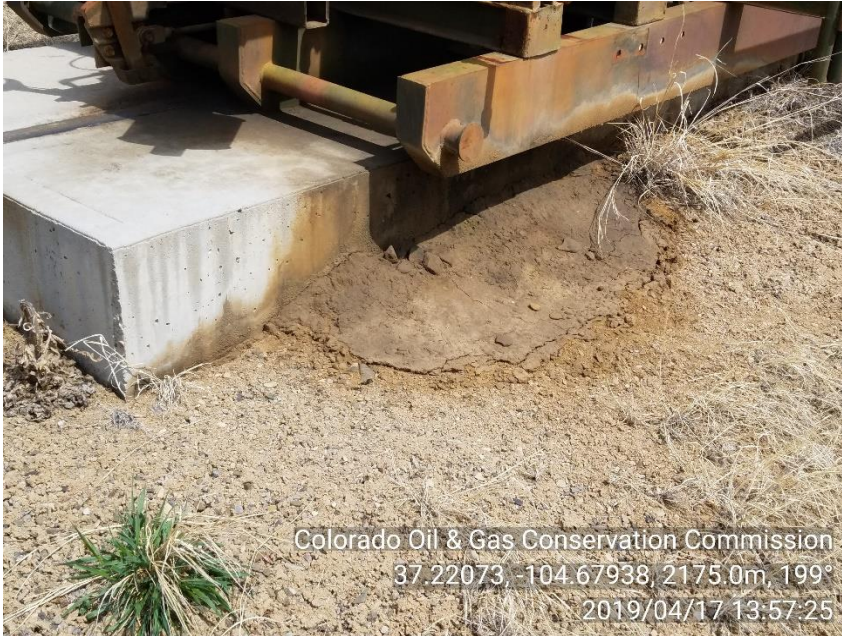
PHOTO 3: IMPACTED SOIL ON NORTHWEST SIDE OF PUMPJACK SKID NEAR PRIME MOVER
