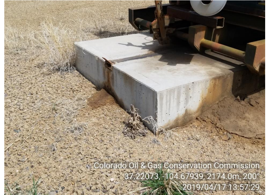
PHOTO 4: IMPACTED SOIL ON NORTH SIDE OF PUMPJACK SKID NEAR PRIME MOVER
