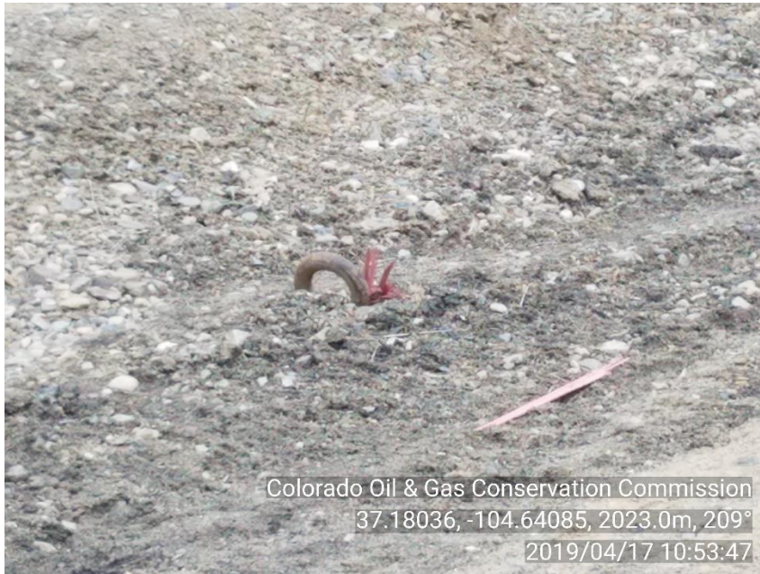
PHOTO 3: NO ANCHOR MARKER
